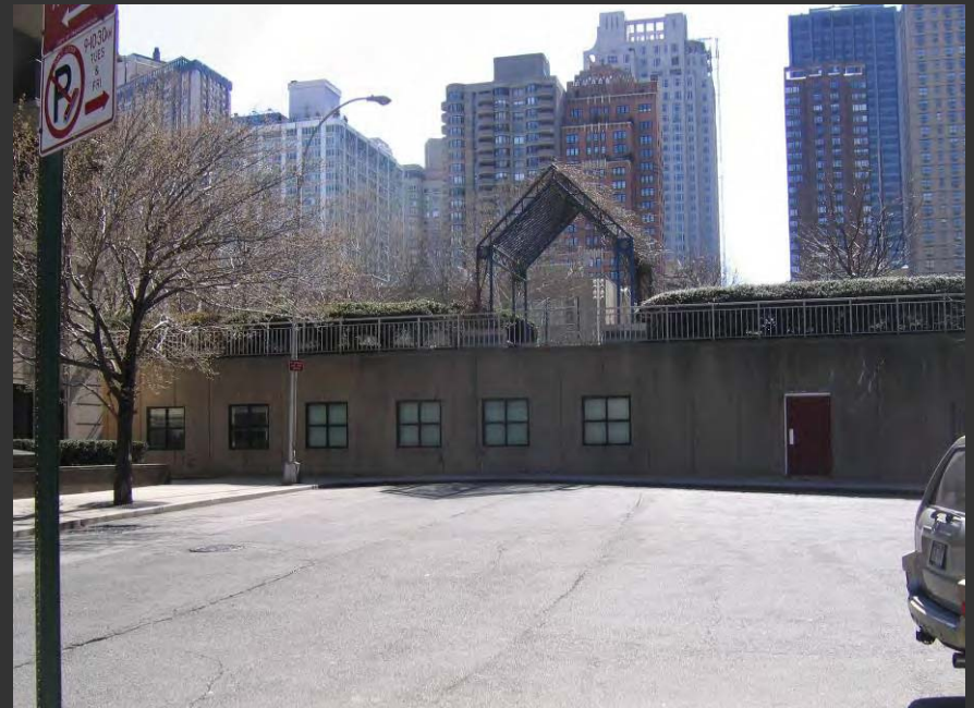
W. 61 st Street Looking East
