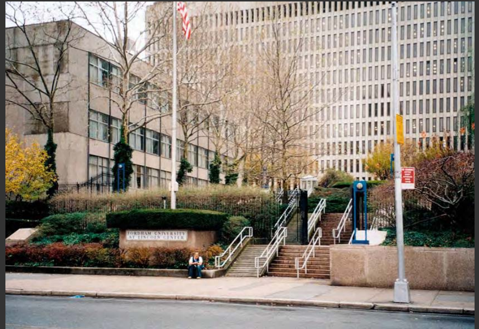
W. 62 nd Street Access to Plaza
