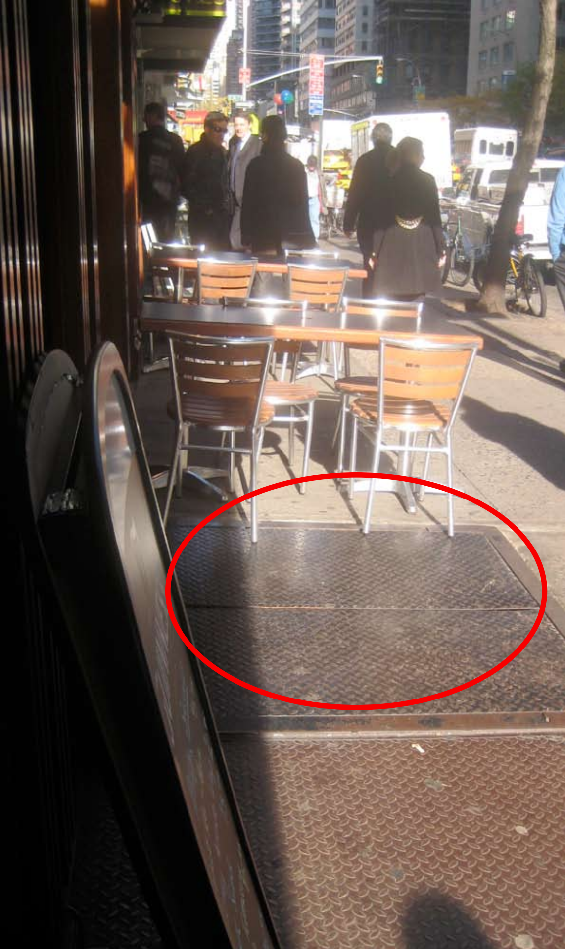
Several times sidewalk cafes place chairs or tables on basement grates which is not permitted. This photo is taken at Pig n' Whistle on 3rd ave
