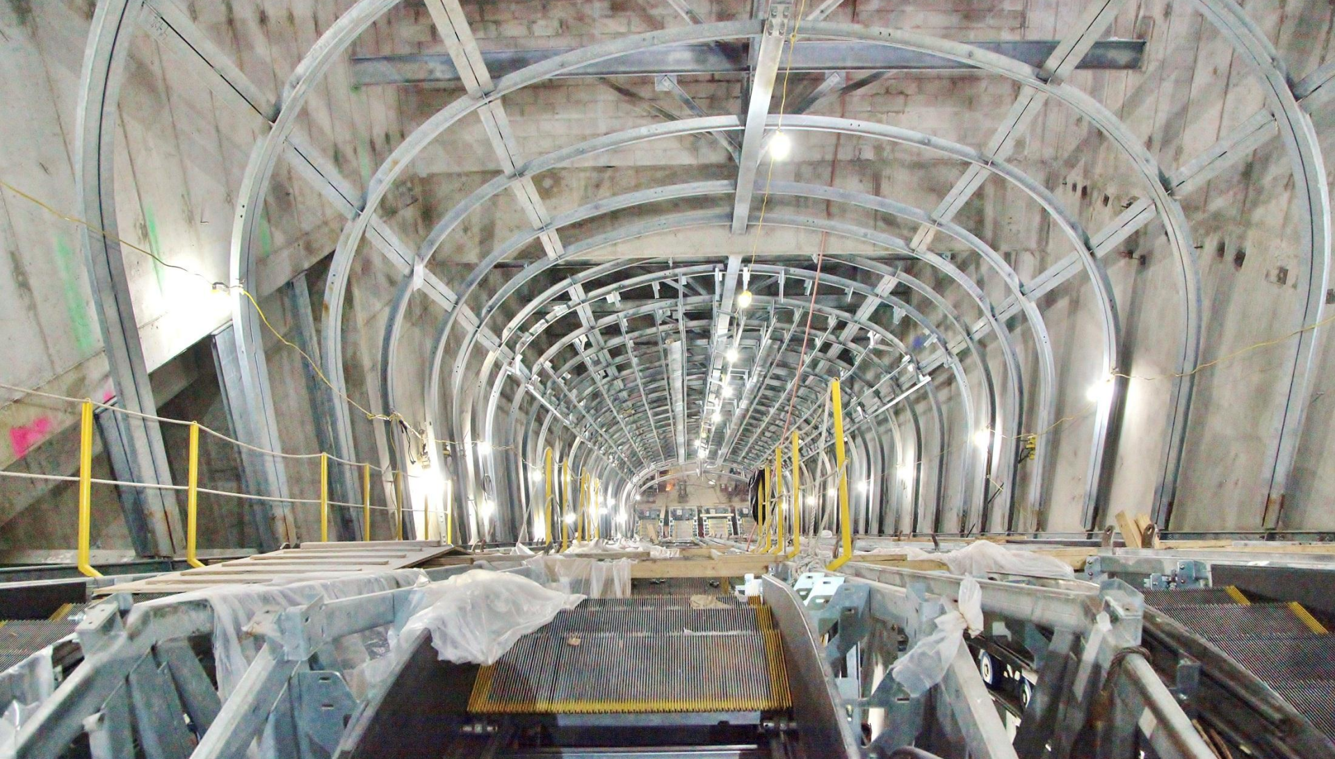
SITE J – E2 TUNNEL – ARCHITECTURAL FINISHES JUNE 2014
