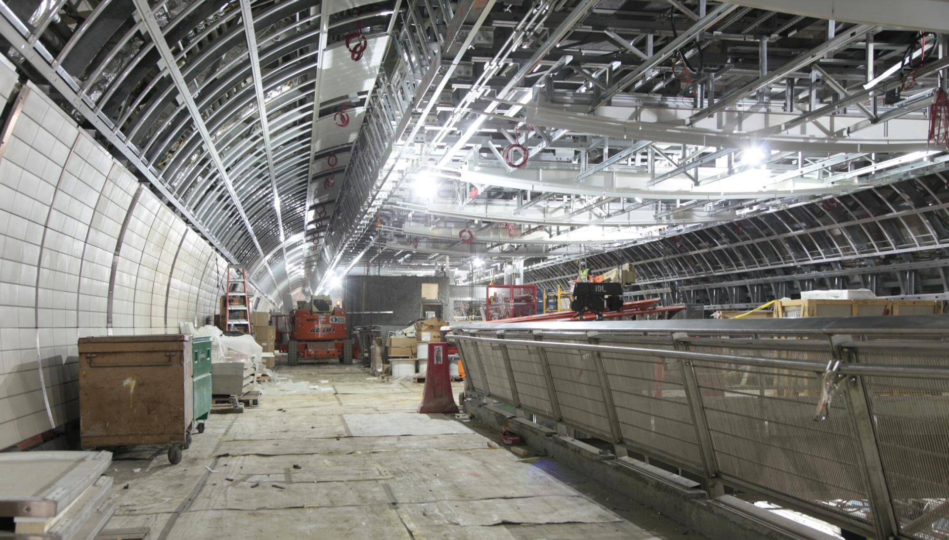
34 TH STREET STATION- LOWER MEZZANINE APRIL 2014
