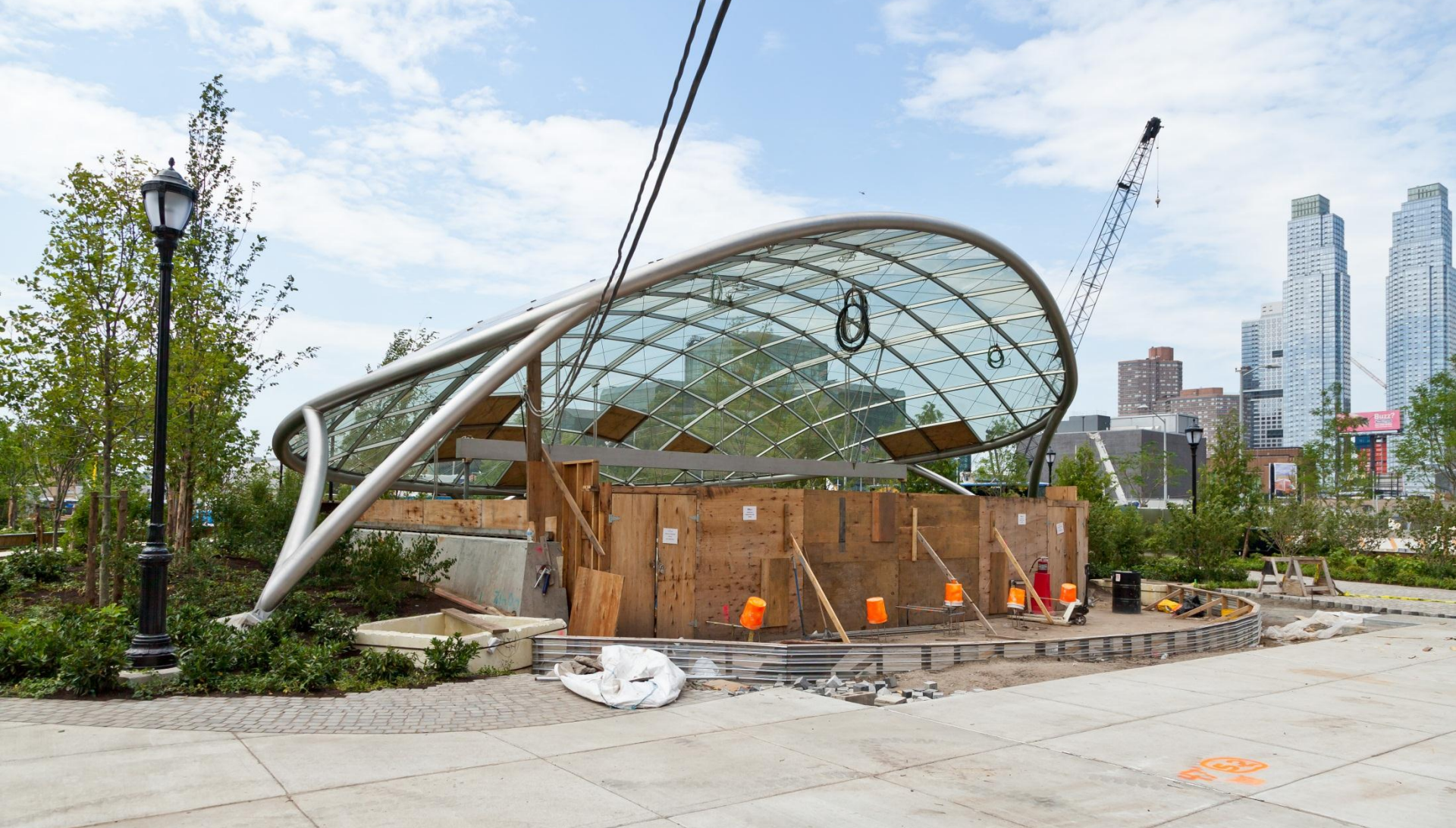
SITE J CANOPY LOOKING WEST ( C-26512) JUNE 2014
