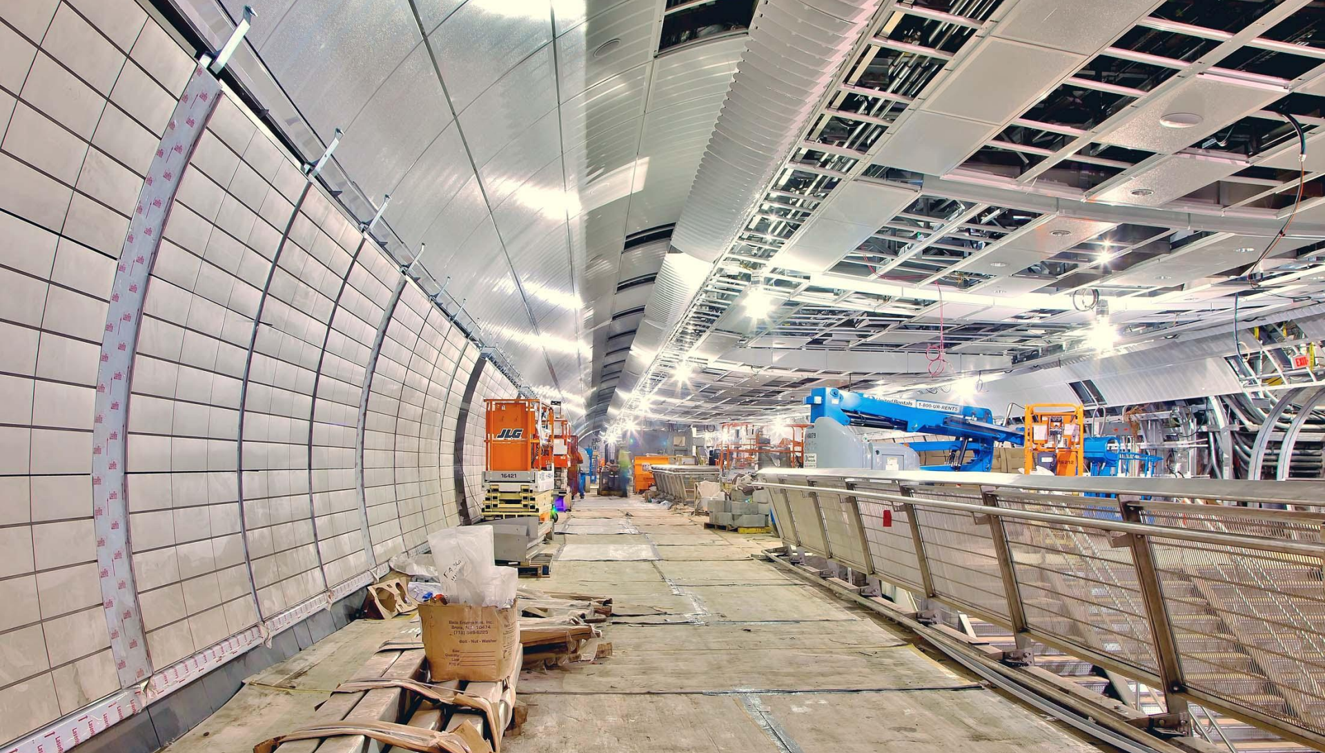
34 TH STREET STATION- LOWER MEZZANINE JUNE 2014
