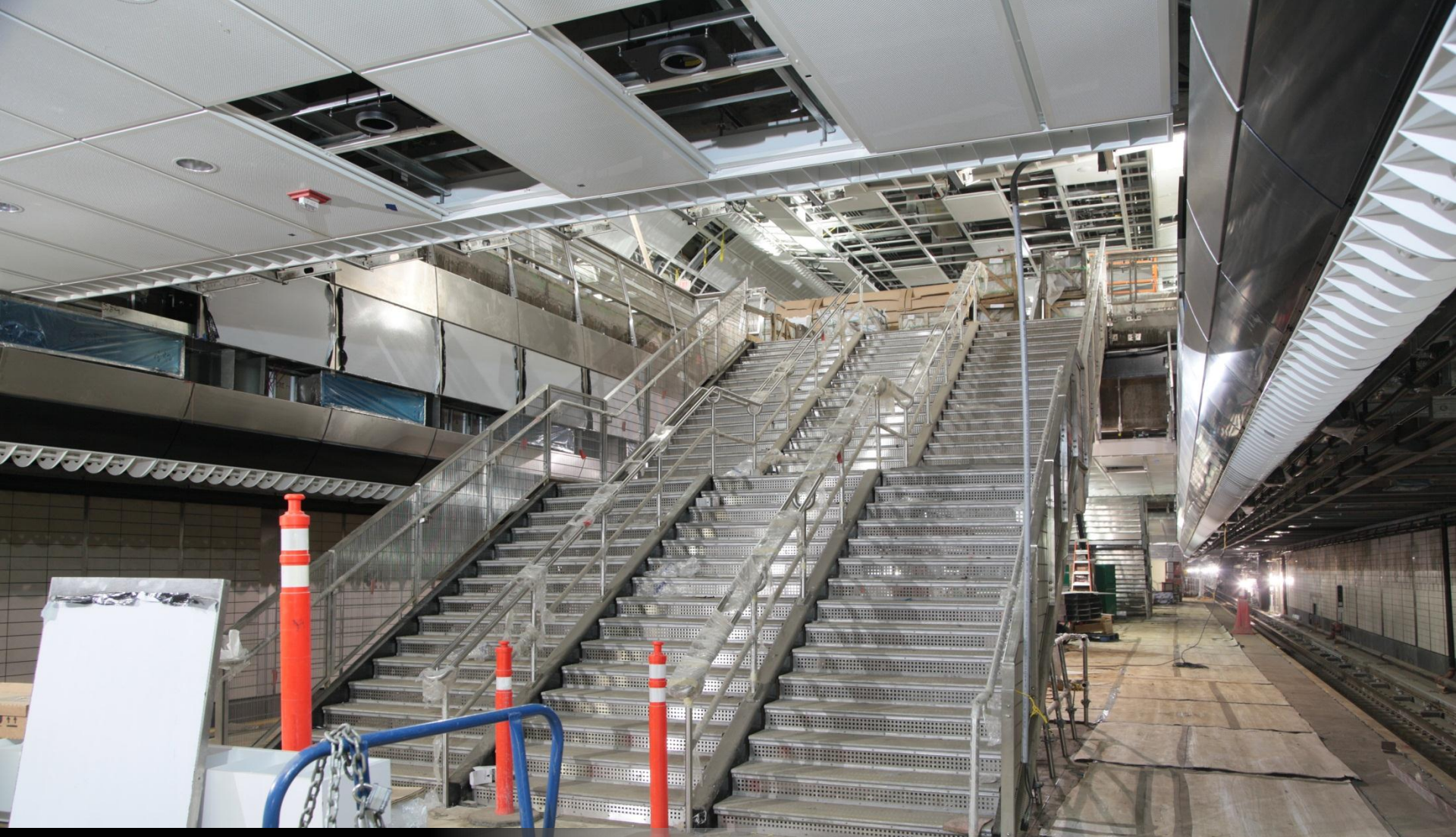
34 TH STREET STATION - PLATFORM LEVEL JUNE 2014
