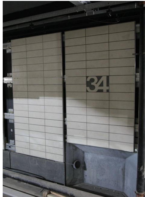
Installing GFRG Sub-Framing and Panels on track wall
