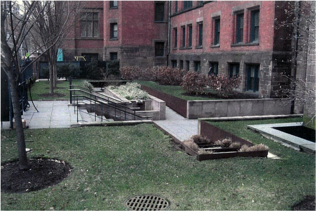
Garden before alteration, and as existing
