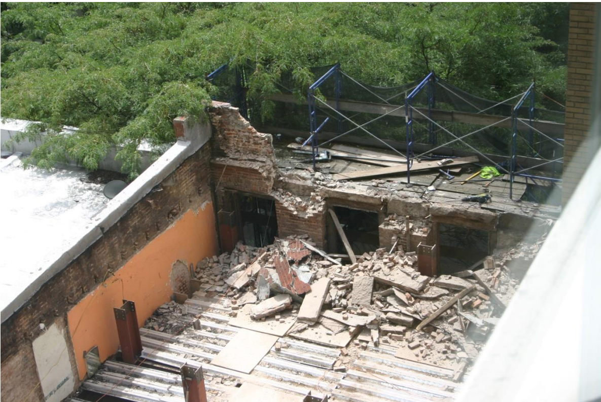
Demolition of façade at 335-337 West 55 th Street
