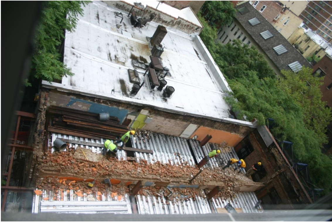
Demolition of party wall between 335 and 337 West 55 th Street
