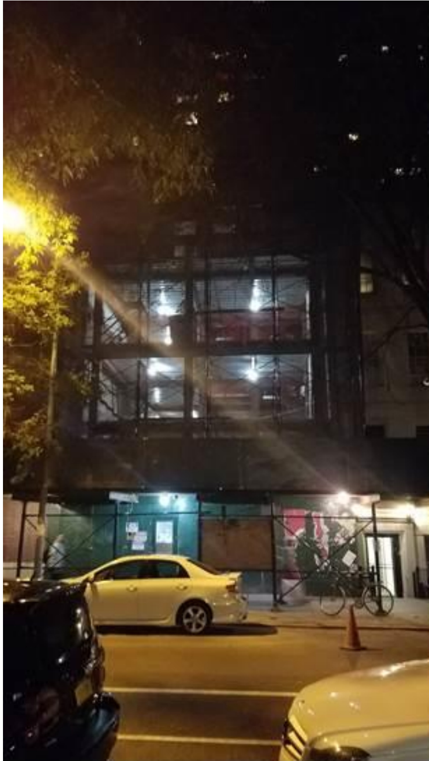
Building façade removed by August 2017
