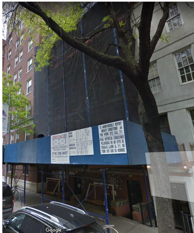
Pipe scaffold and sidewalk bridge installed by May 2016. Source: Google Streetview
