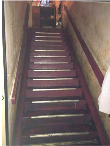
STAIRS TO FIRST FLOOR
