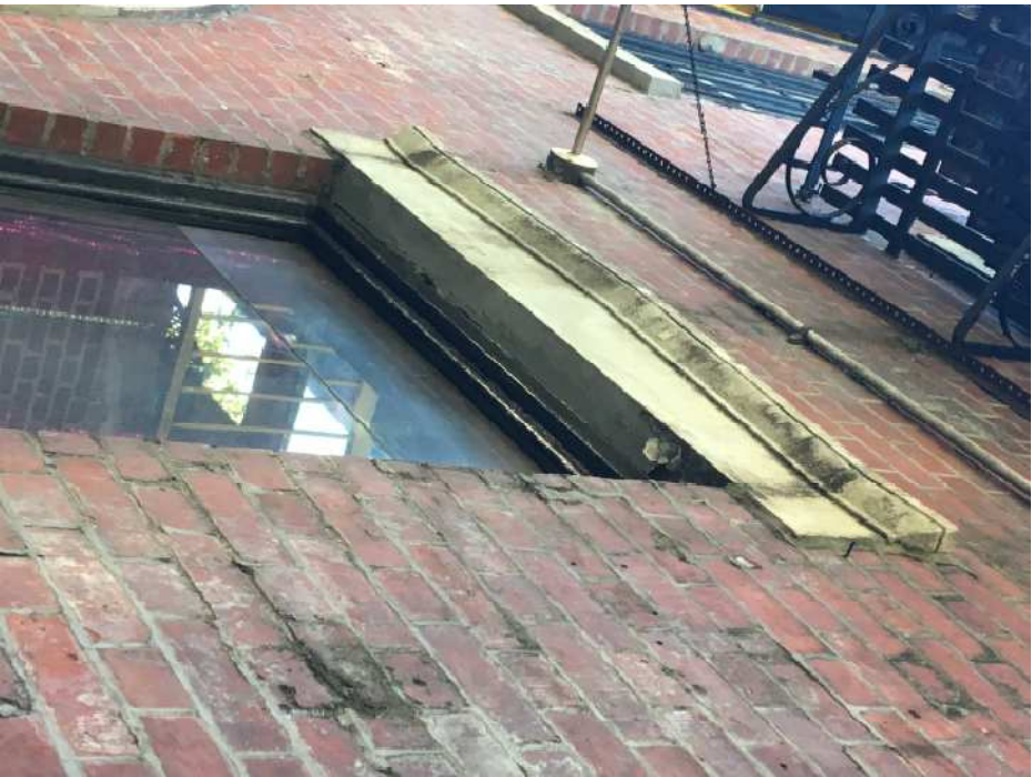
Condition of brick and marble lintels
