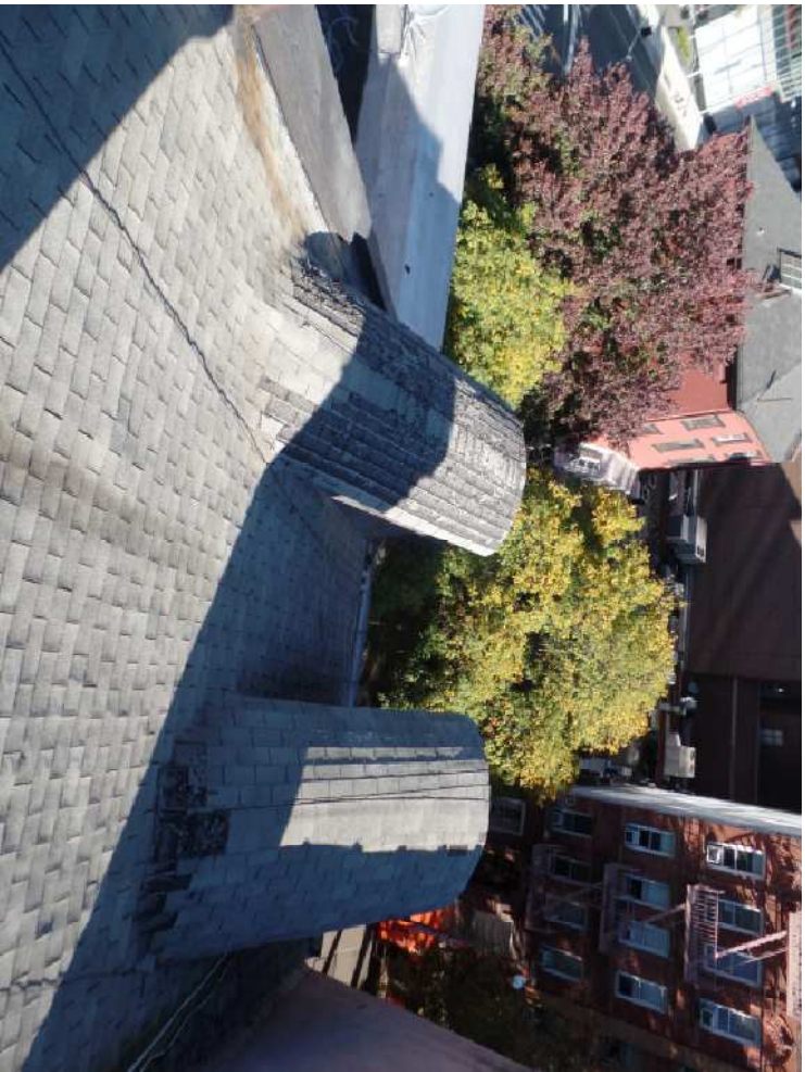
Asphalt shingles at front roof and dormers
