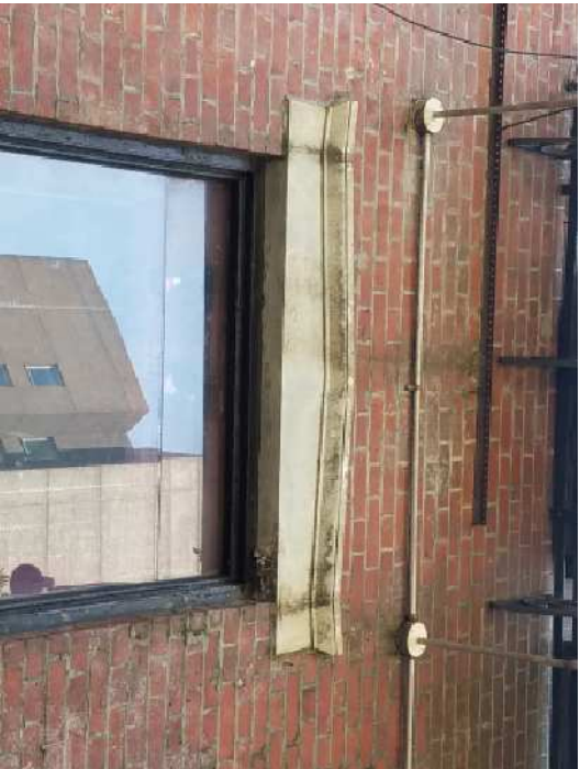
Condition of brick and marble lintels
