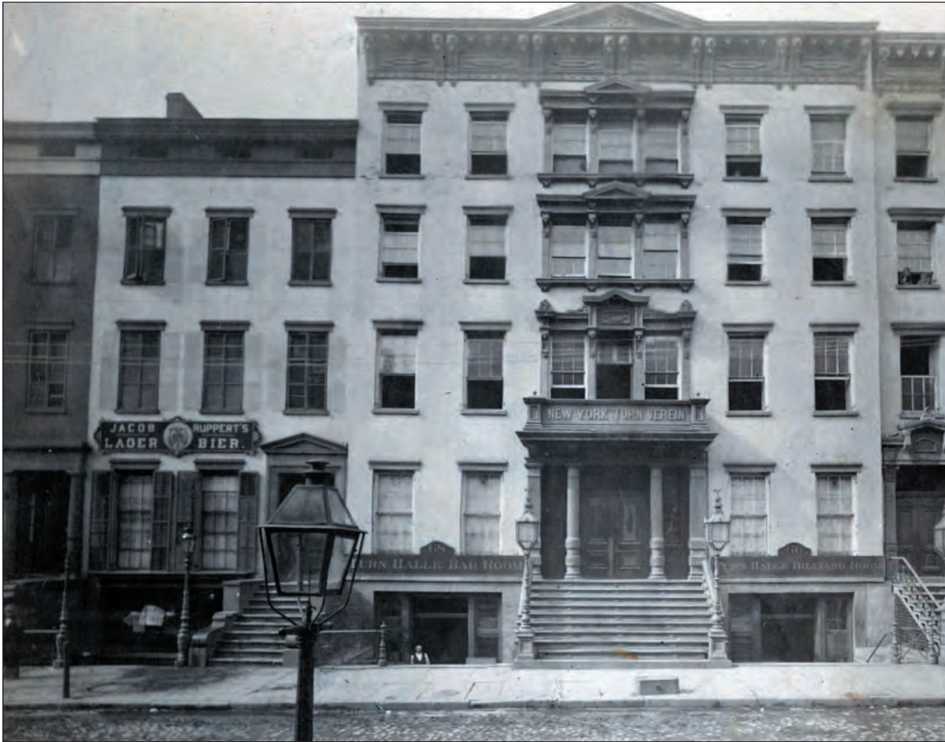
No. 70 East 4th Street ca. 1875, first full building from the left. The only alterations to the original building appear to be the basement storefront, “Jacob Ruppert’s Lager Bier” sign, and possibly paint on the brick façade. The New York Turn Verein occupies the two center projecting buildings, nos. 66-68, which have been more extensively modified.
