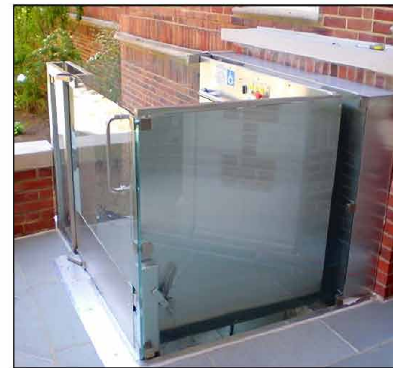
TYPICAL EXTERIOR LIFT
