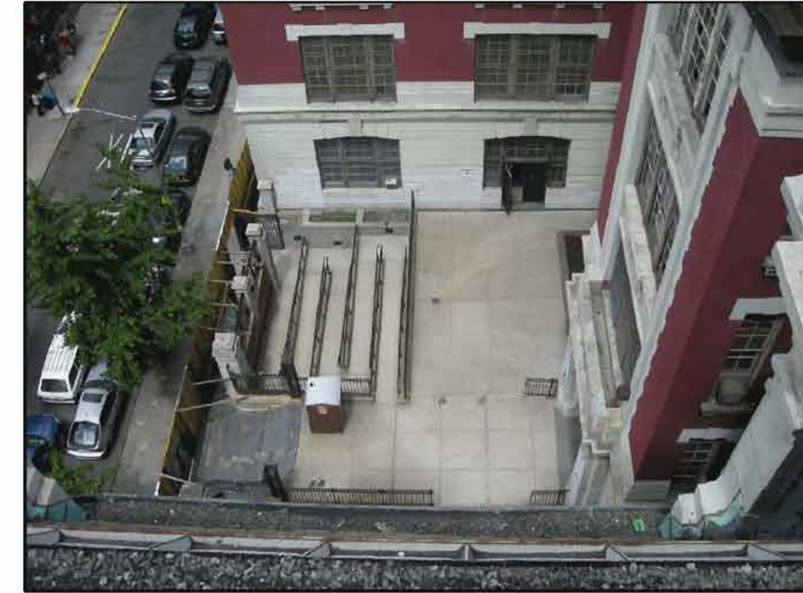
9TH STREET PHOTO - COURTYARD VIEW FROM ROOF
