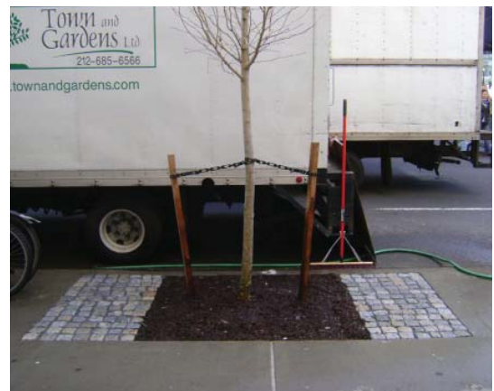
The completed tree pit.
