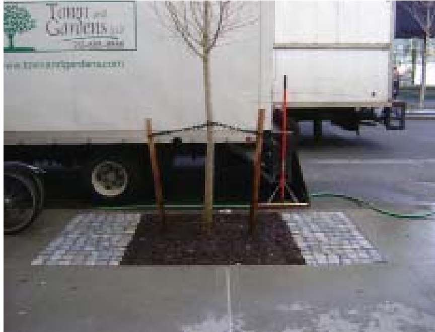
Cobble pavers, set in sand bed. New tree planting.
