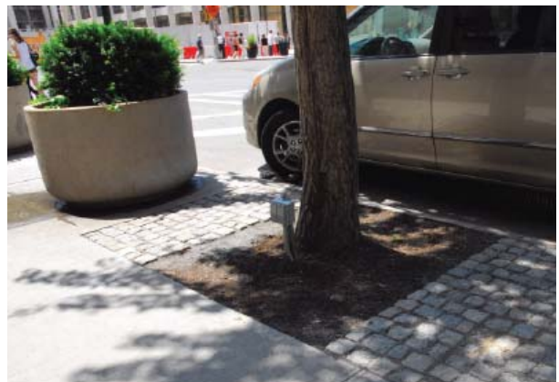
Existing tree pit expanded. Cobble pavers, set in sand bed, around existing trees.
