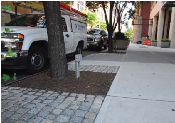
Existing tree pit expanded. Cobble pavers, set in sand bed, around existing trees.
