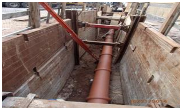
ALAMO PLAZA: NEWLY INSTALLED 15" SEWER MAIN PIPE
