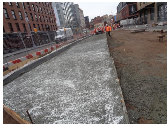
Placement of Road Base on 9 th Avenue
