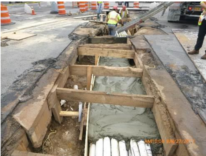
Con Edison Duct Installation in Progress - Concrete Pour
