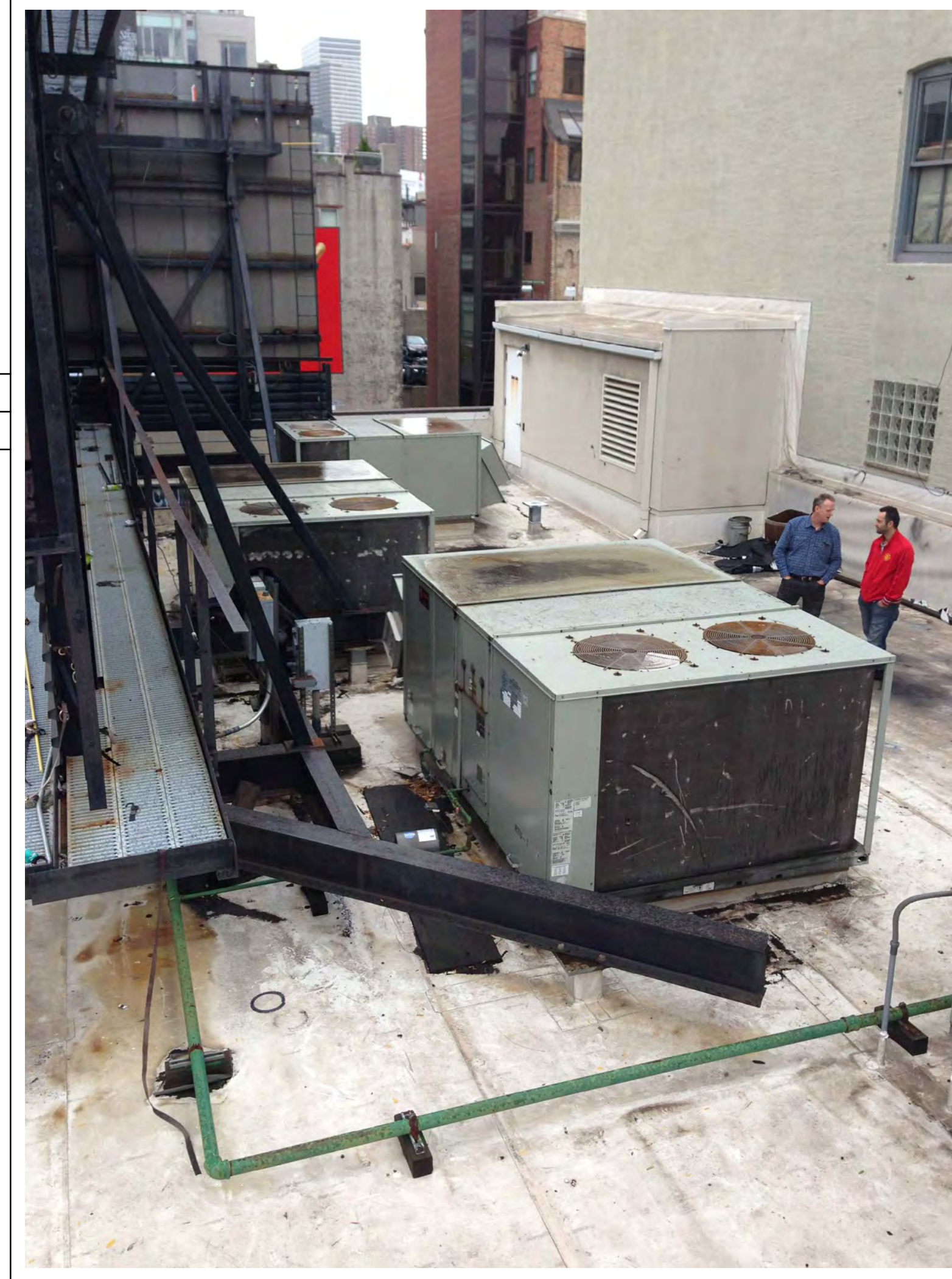
5 SOUTHWEST ROOF VIEW FROM NORTHEAST CORNER SCALE: NOT TO SCALE
