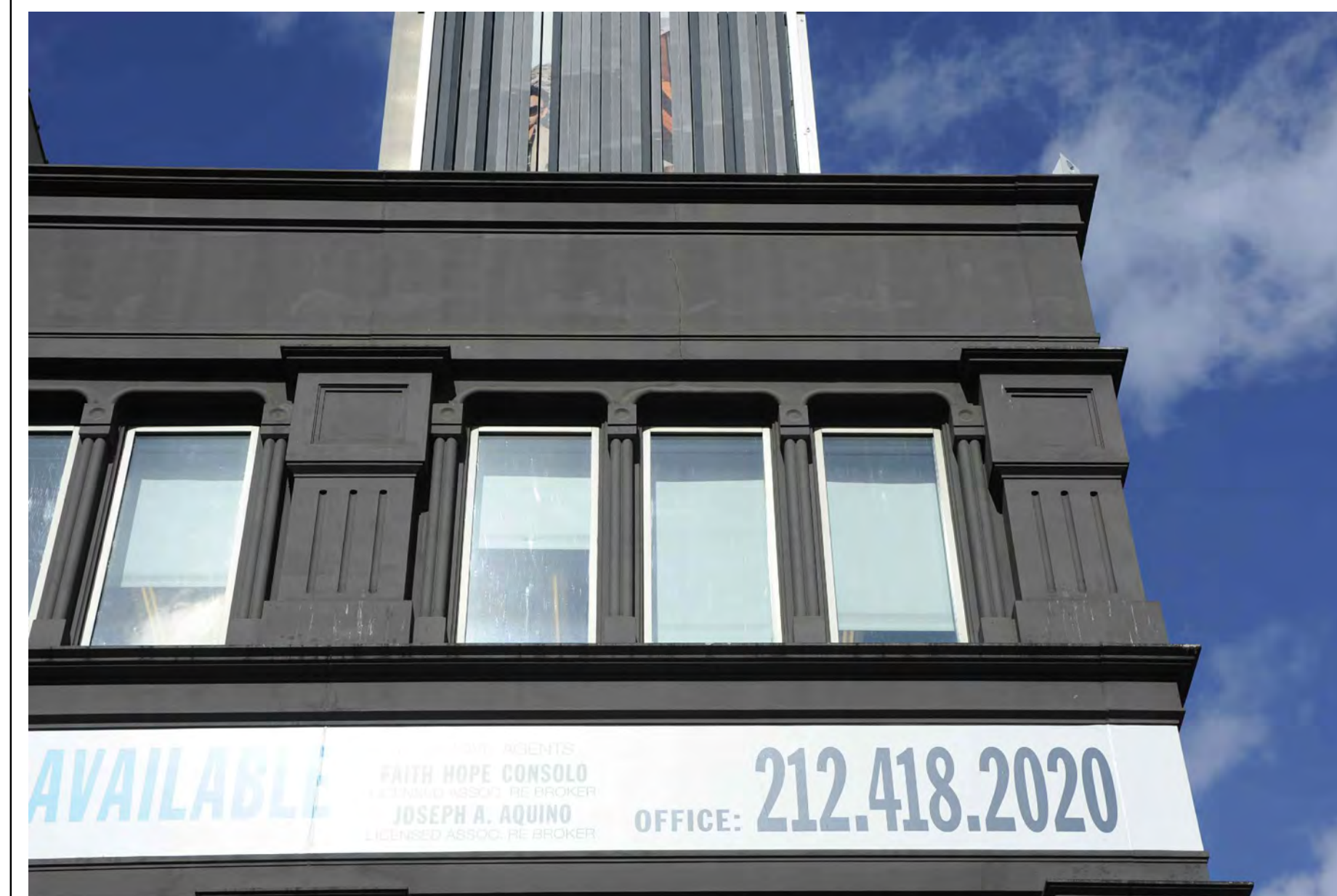
2 EXISTING CONDITIONS: BROOME STREET FACADE CLOSE-UP SCALE: NOT TO SCALE
