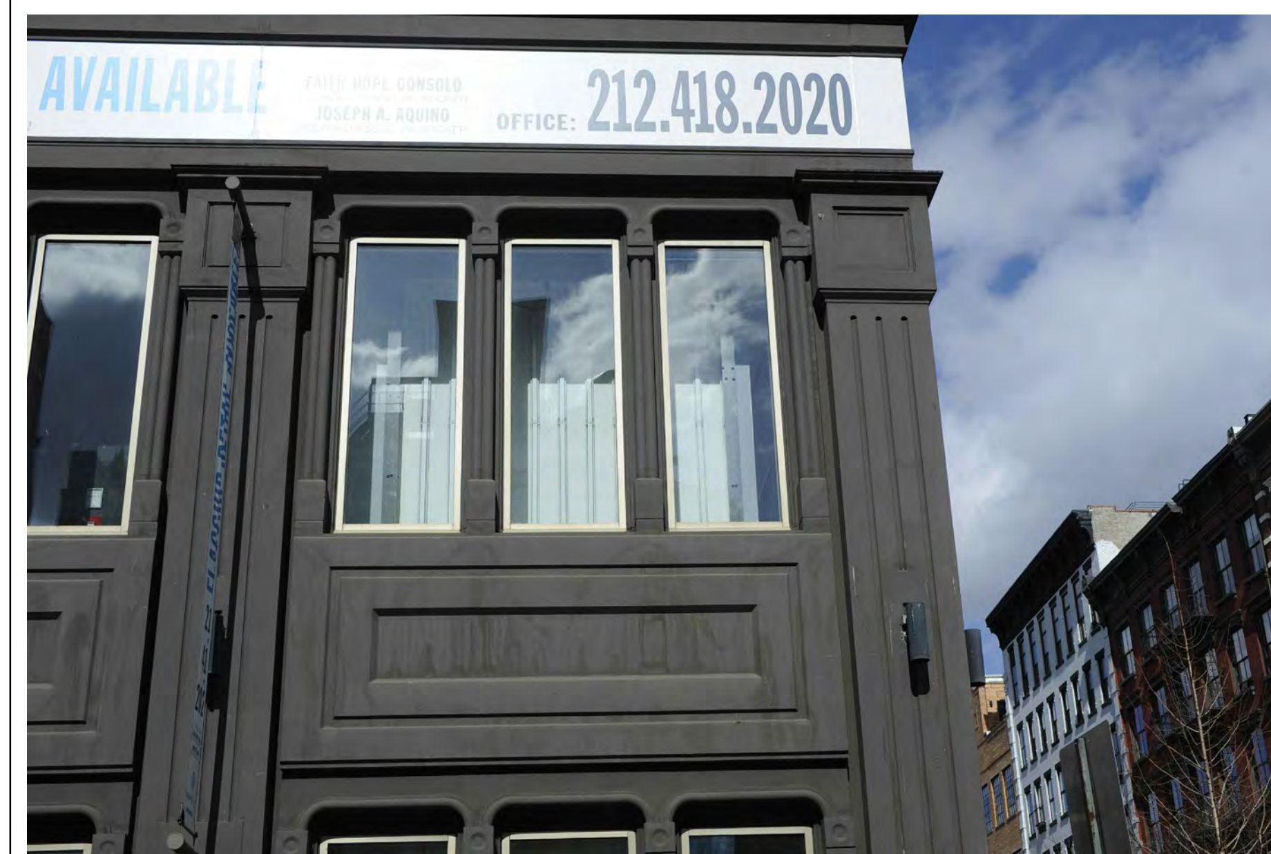
4 EXISTING CONDITIONS: BROOME STREET FACADE CLOSE-UP SCALE: NOT TO SCALE
