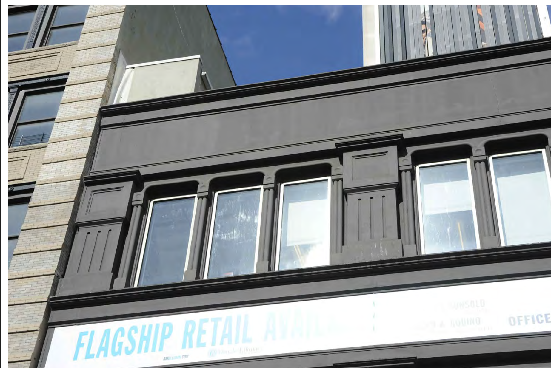
1 EXISTING CONDITIONS: BROOME STREET FACADE CLOSE-UP SCALE: NOT TO SCALE
