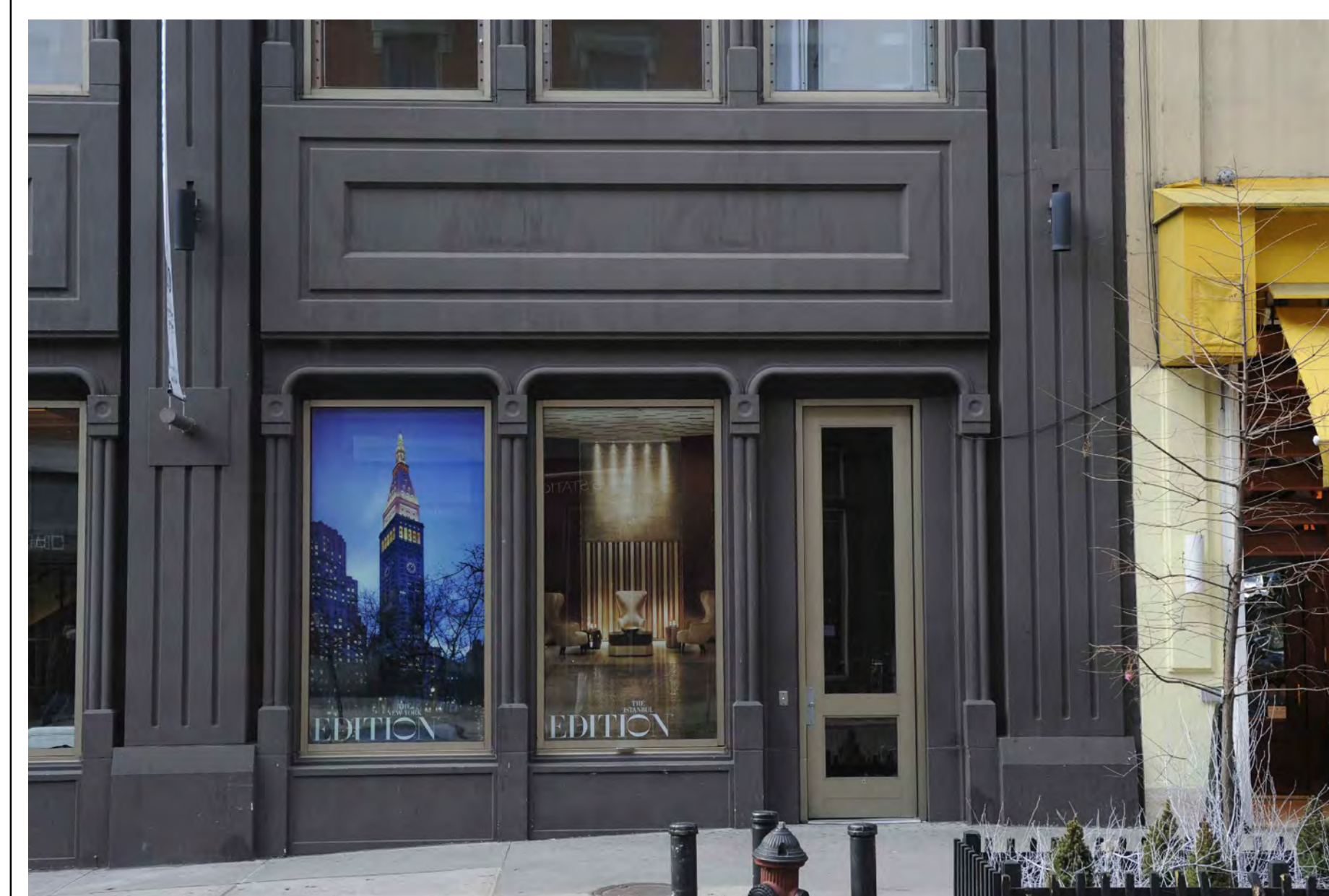
9 EXISTING CONDITIONS: WEST BROADWAY FACADE CLOSE-UP SCALE: NOT TO SCALE
