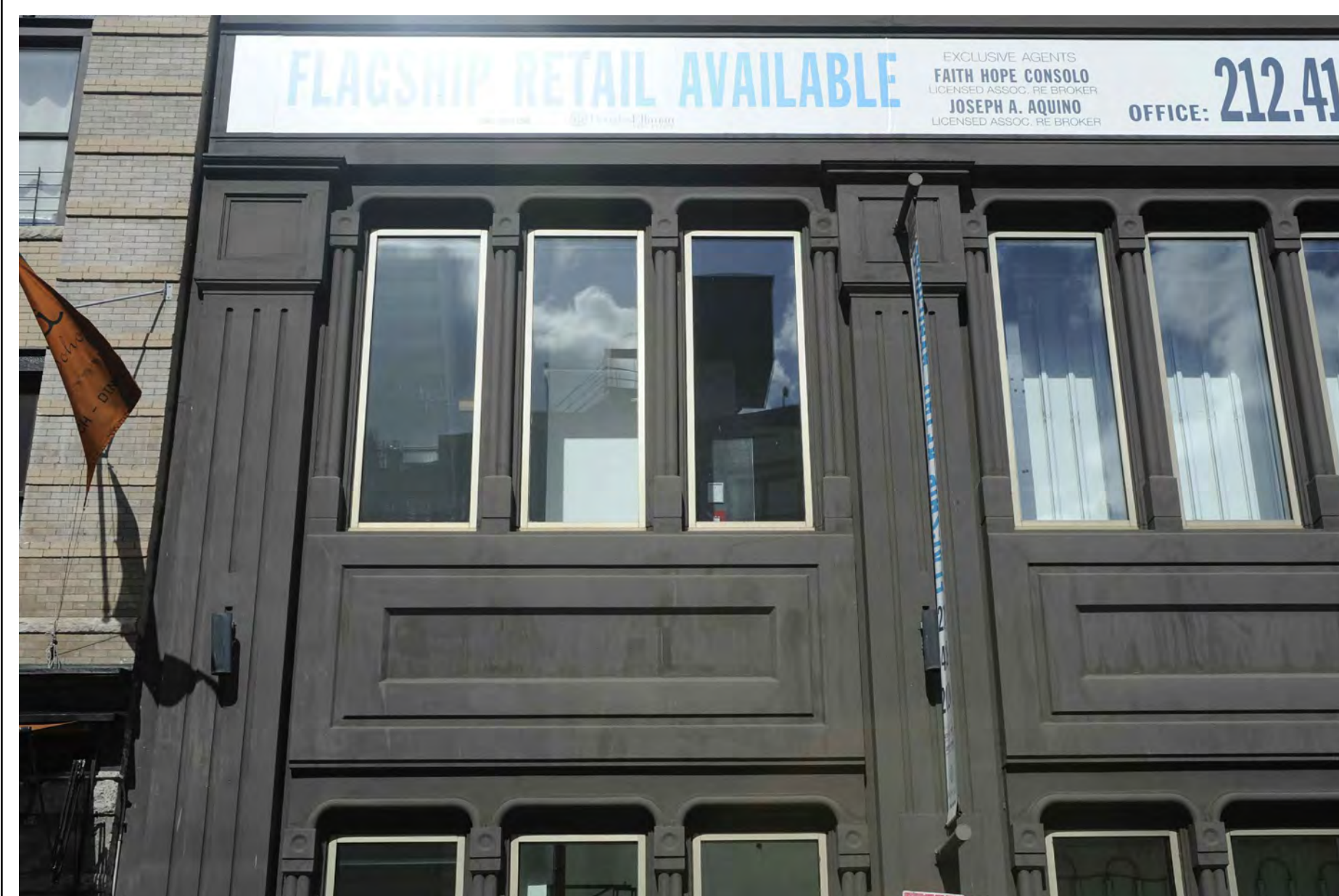
3 EXISTING CONDITIONS: BROOME STREET FACADE CLOSE-UP SCALE: NOT TO SCALE
