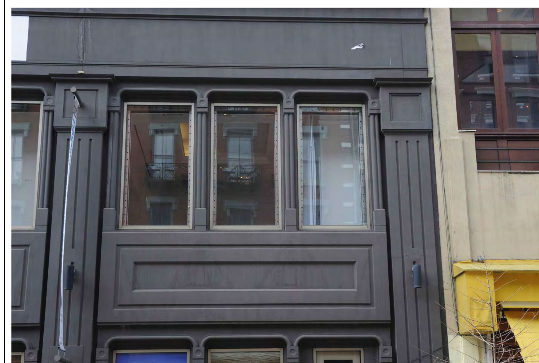
6 EXISTING CONDITIONS: WEST BROADWAY FACADE CLOSE-UP SCALE: NOT TO SCALE
