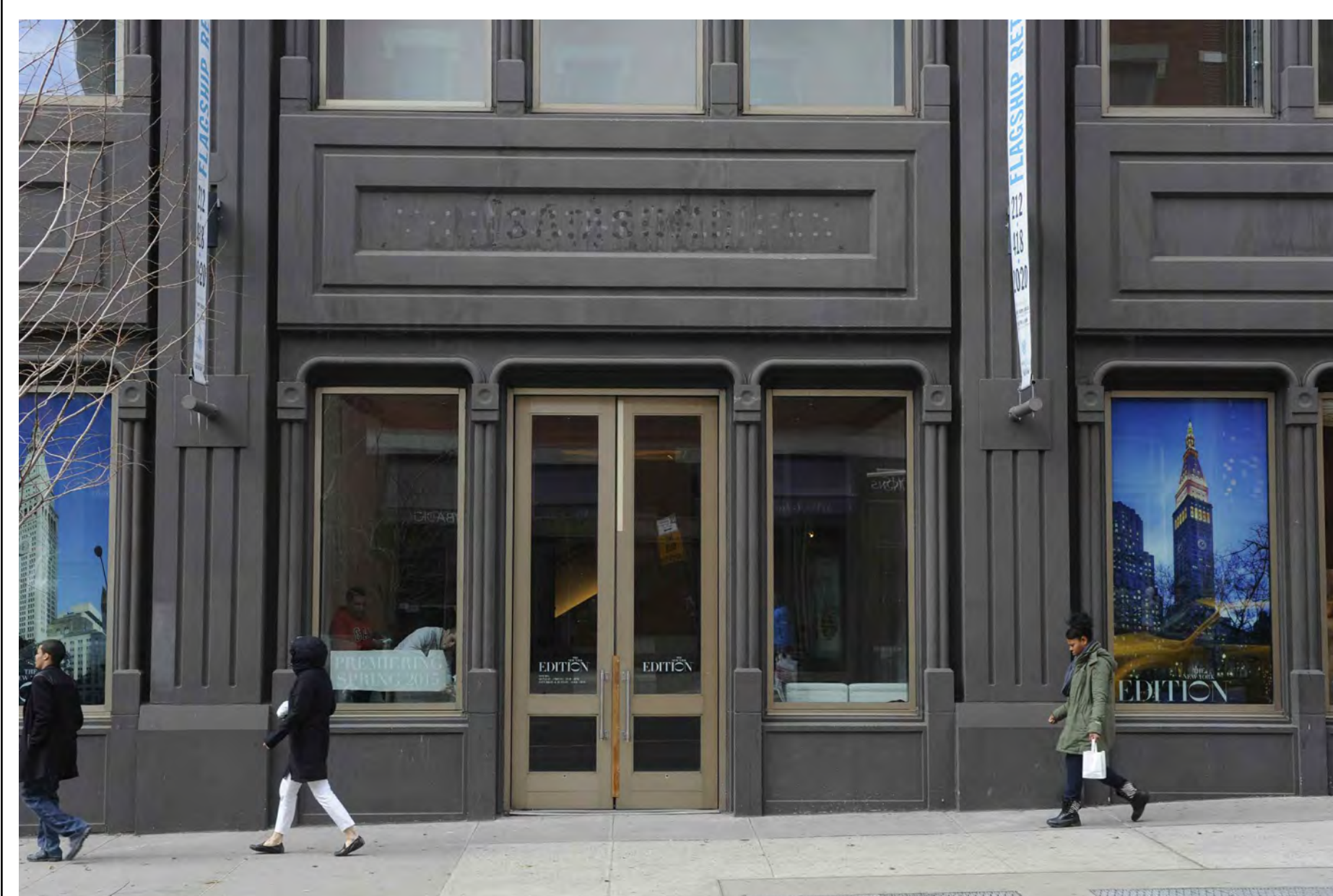
8 EXISTING CONDITIONS: WEST BROADWAY FACADE CLOSE-UP SCALE: NOT TO SCALE
