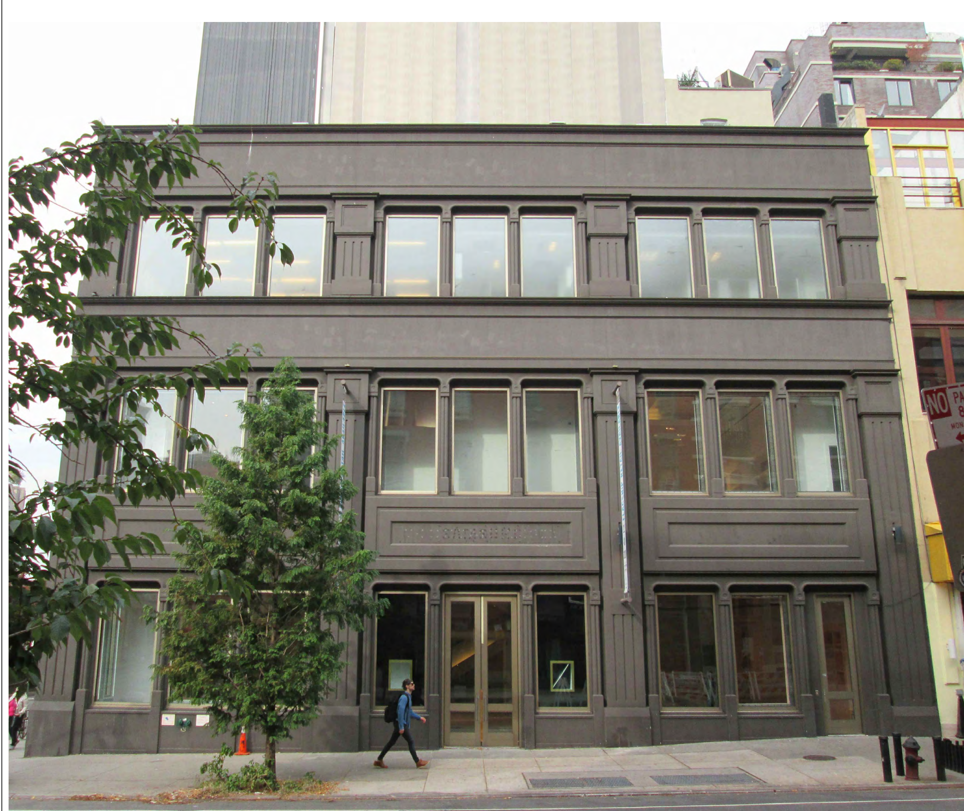
2 EXISTING CONDITIONS OF 374 WEST BROADWAY: WEST BROADWAY FACADE SCALE: NOT TO SCALE
