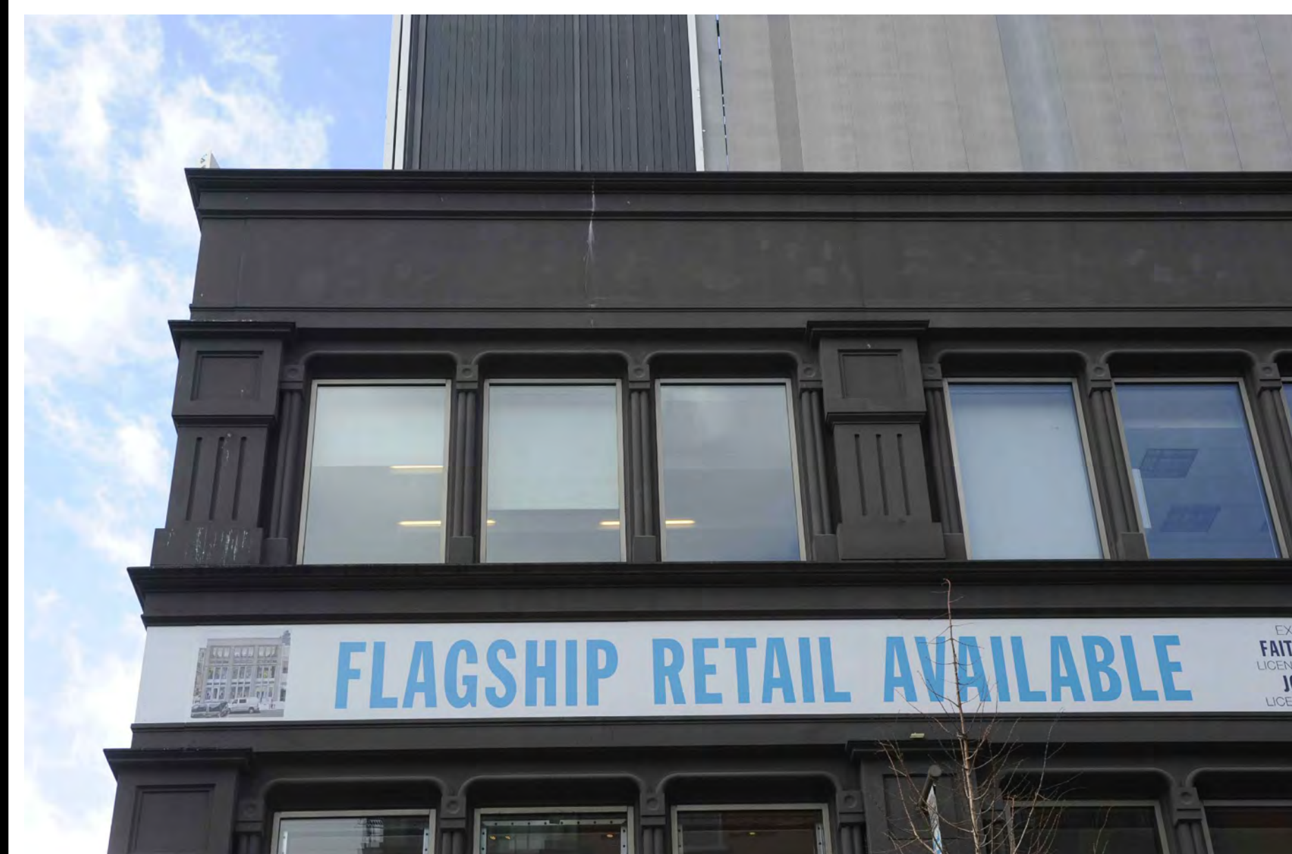
1 EXISTING CONDITIONS: WEST BROADWAY FACADE CLOSE-UP SCALE: NOT TO SCALE
