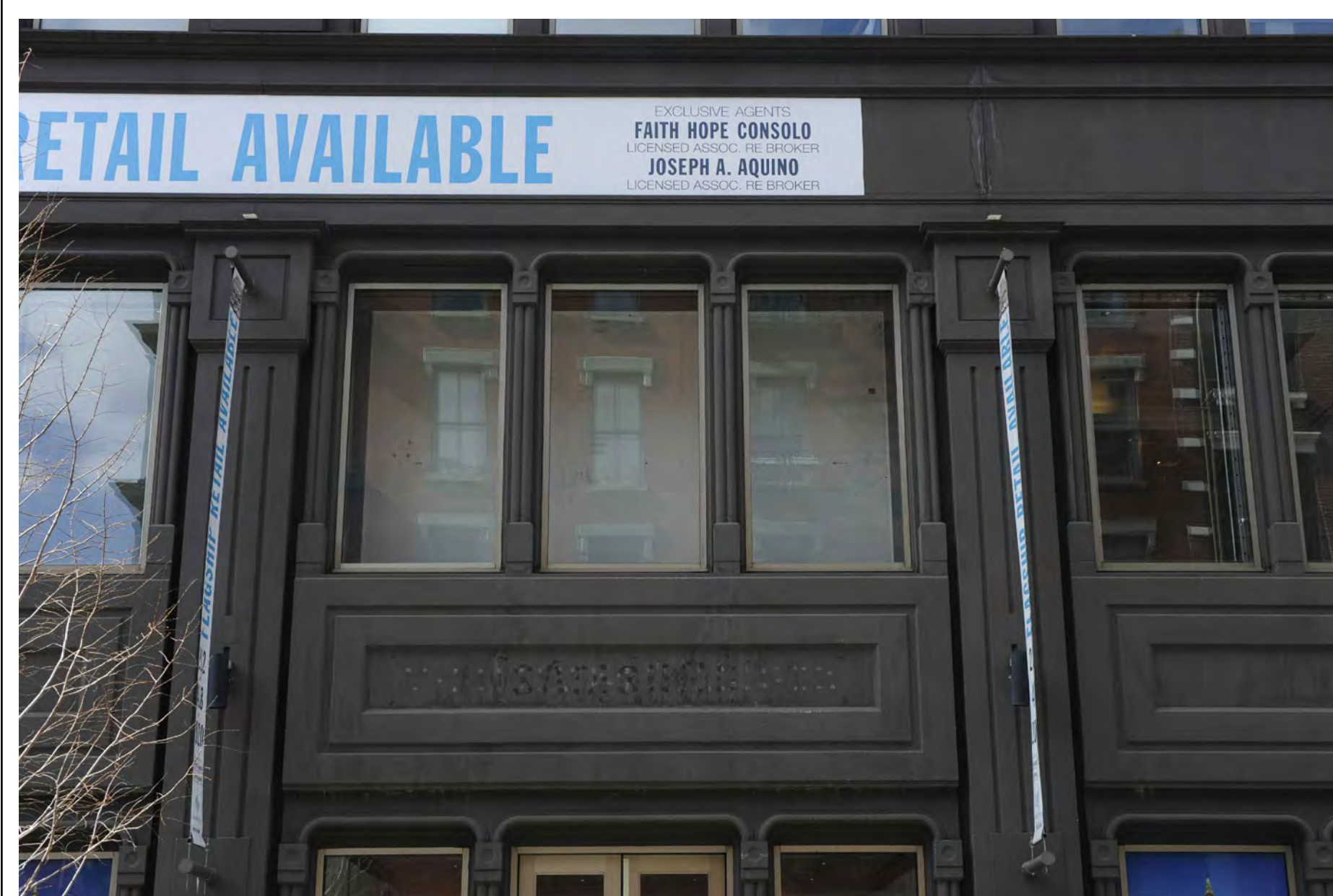
5 EXISTING CONDITIONS: WEST BROADWAY FACADE CLOSE-UP SCALE: NOT TO SCALE
