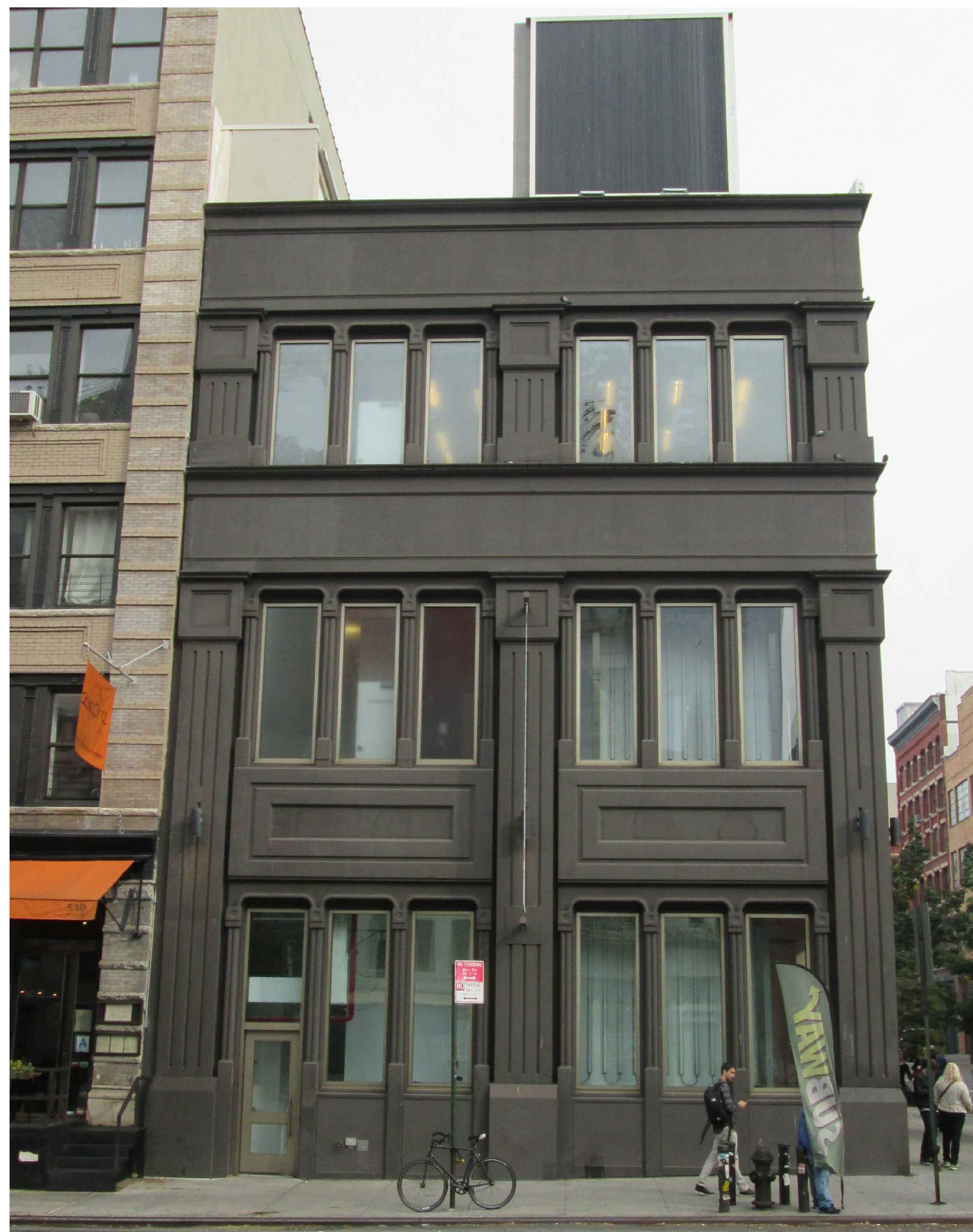
1 EXISTING CONDITIONS OF 374 WEST BROADWAY: BROOME STREET FACADE SCALE: NOT TO SCALE
