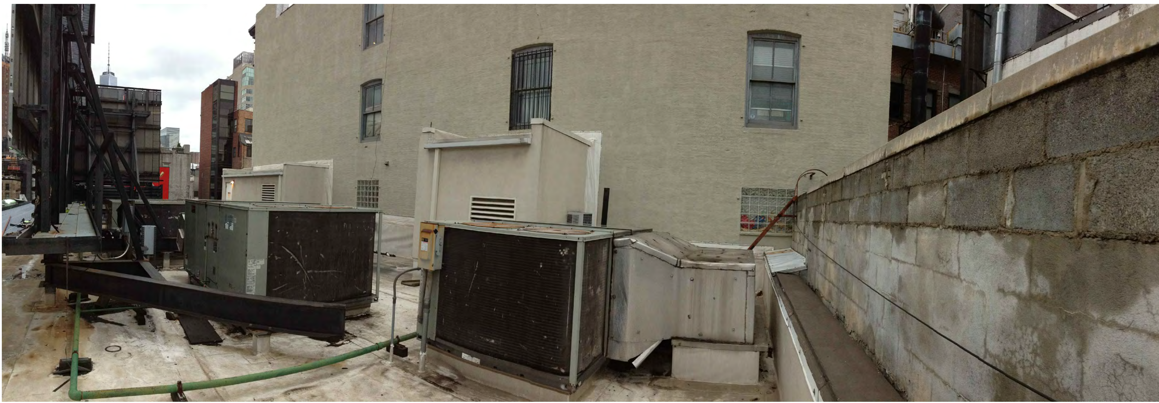
1 EXISTING ROOF CONDITIONS OF 374 WEST BROADWAY: WESTERN VIEW FROM THE NORTHEAST CORNER SCALE: NOT TO SCALE
