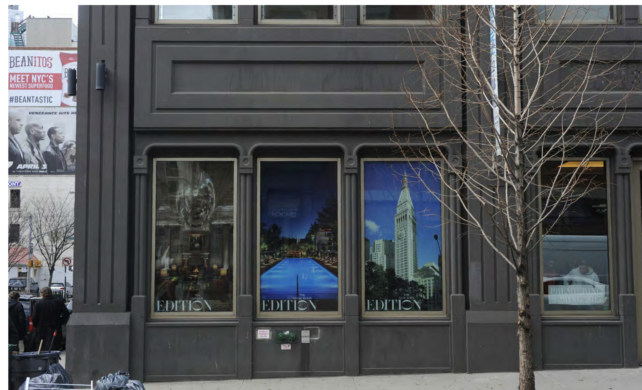
3 EXISTING CONDITIONS OF 374 WEST BROADWAY: SIDEWALK IN AREA OF PROPOSED RAMP SCALE: NOT TO SCALE
