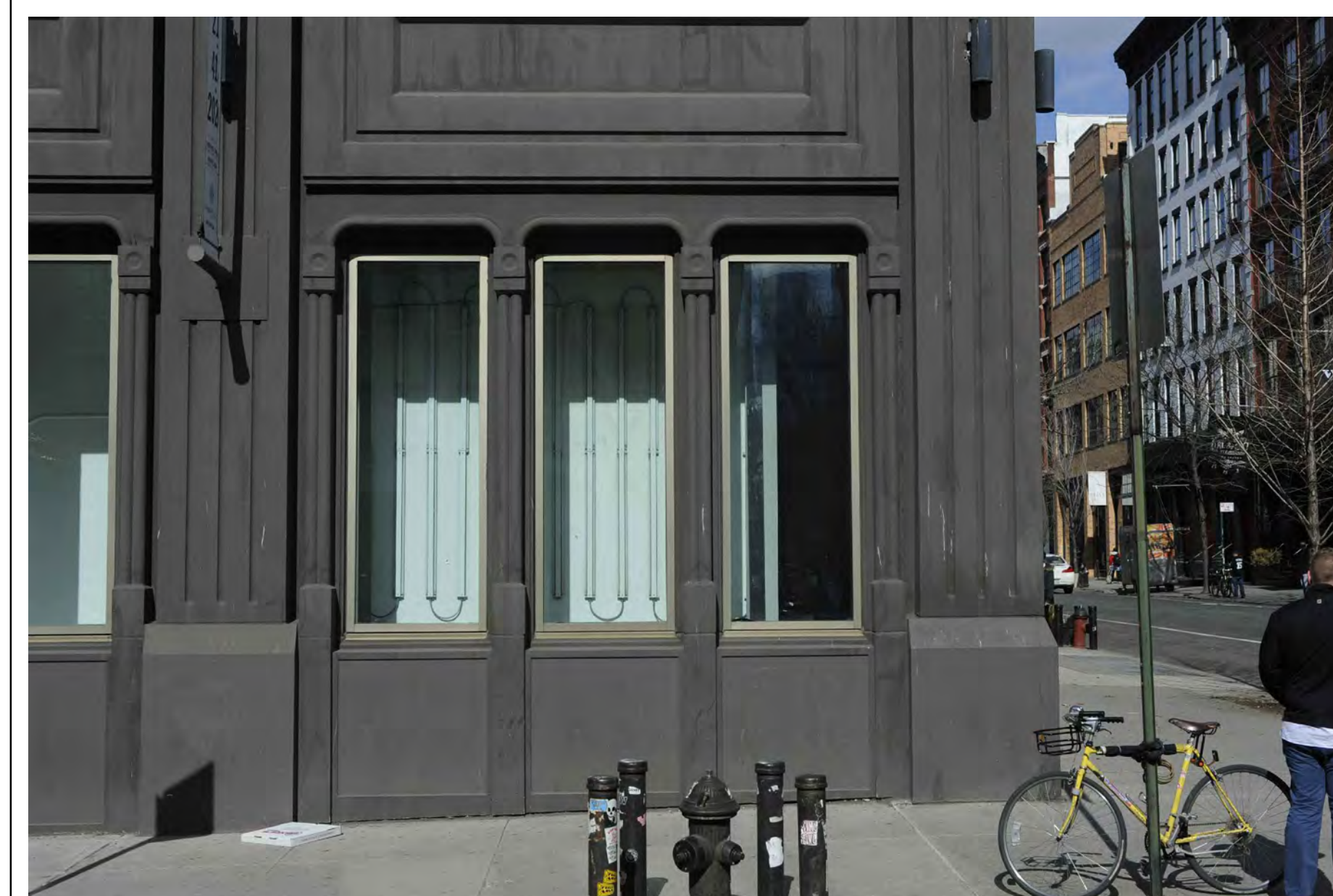
6 EXISTING CONDITIONS: BROOME STREET FACADE CLOSE-UP SCALE: NOT TO SCALE
