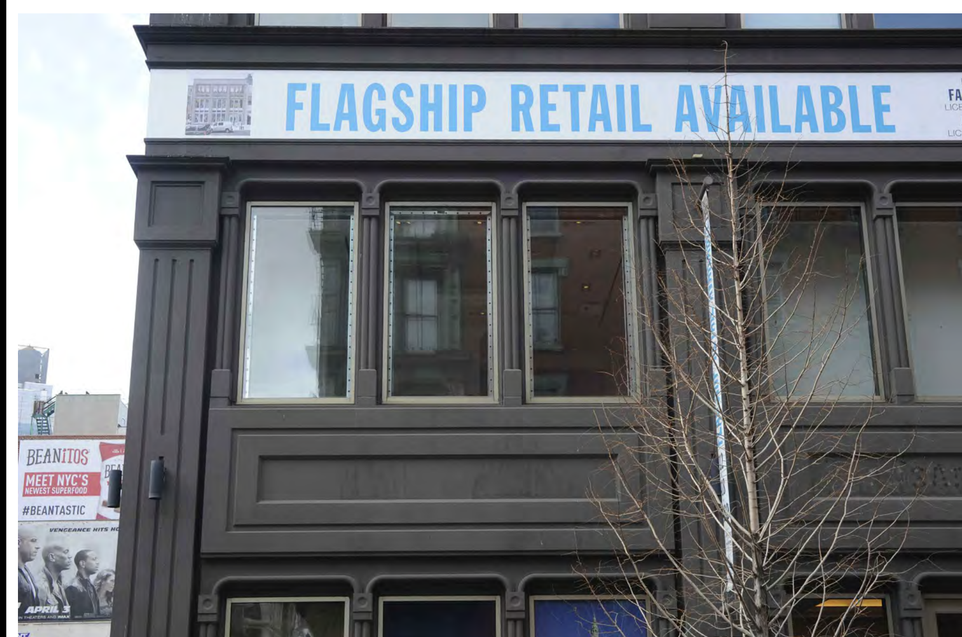
4 EXISTING CONDITIONS: WEST BROADWAY FACADE CLOSE-UP SCALE: NOT TO SCALE
