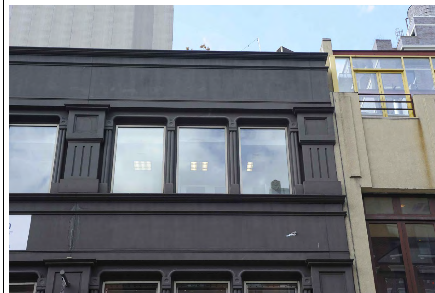
3 EXISTING CONDITIONS: WEST BROADWAY FACADE CLOSE-UP SCALE: NOT TO SCALE
