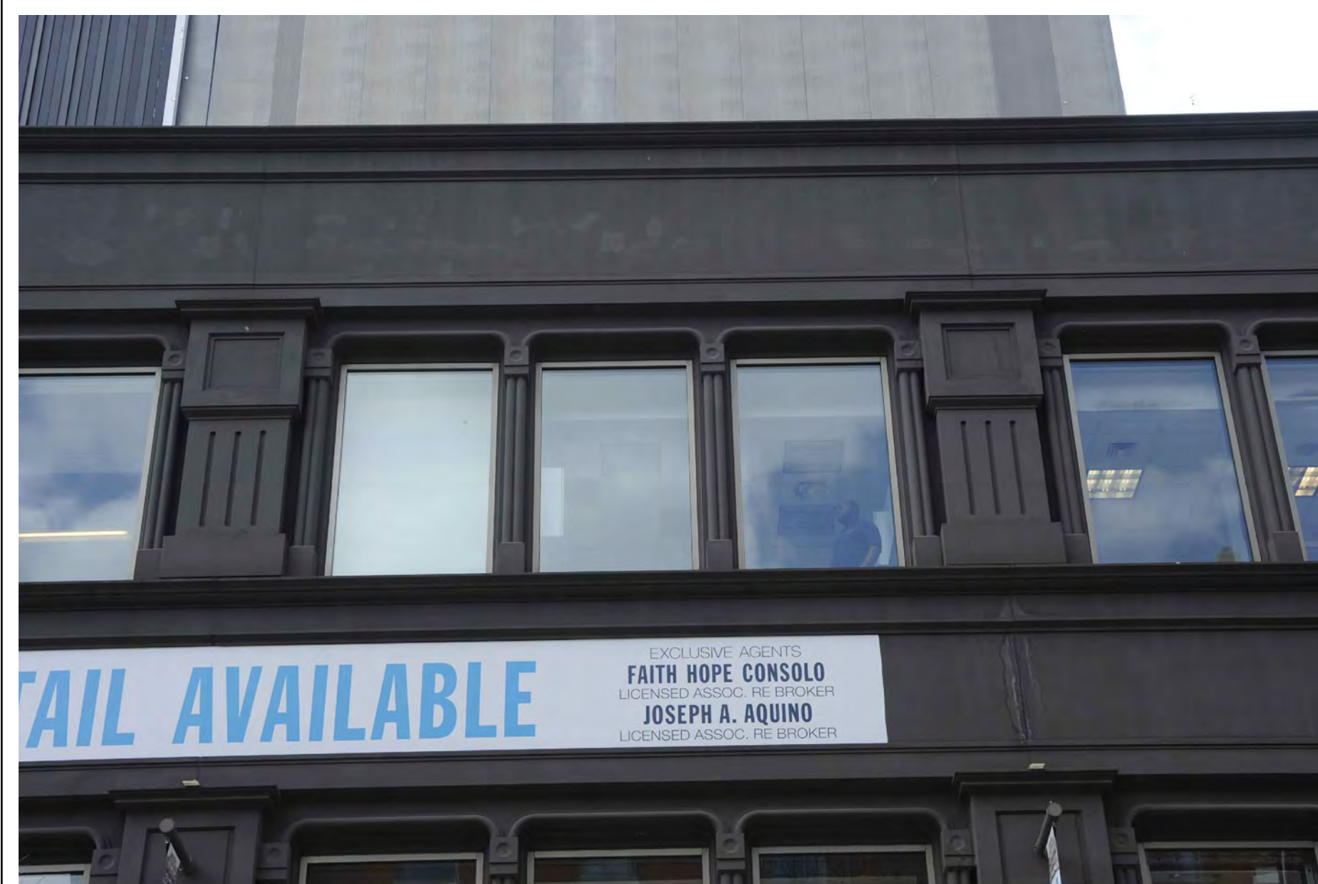
2 EXISTING CONDITIONS: WEST BROADWAY FACADE CLOSE-UP SCALE: NOT TO SCALE
