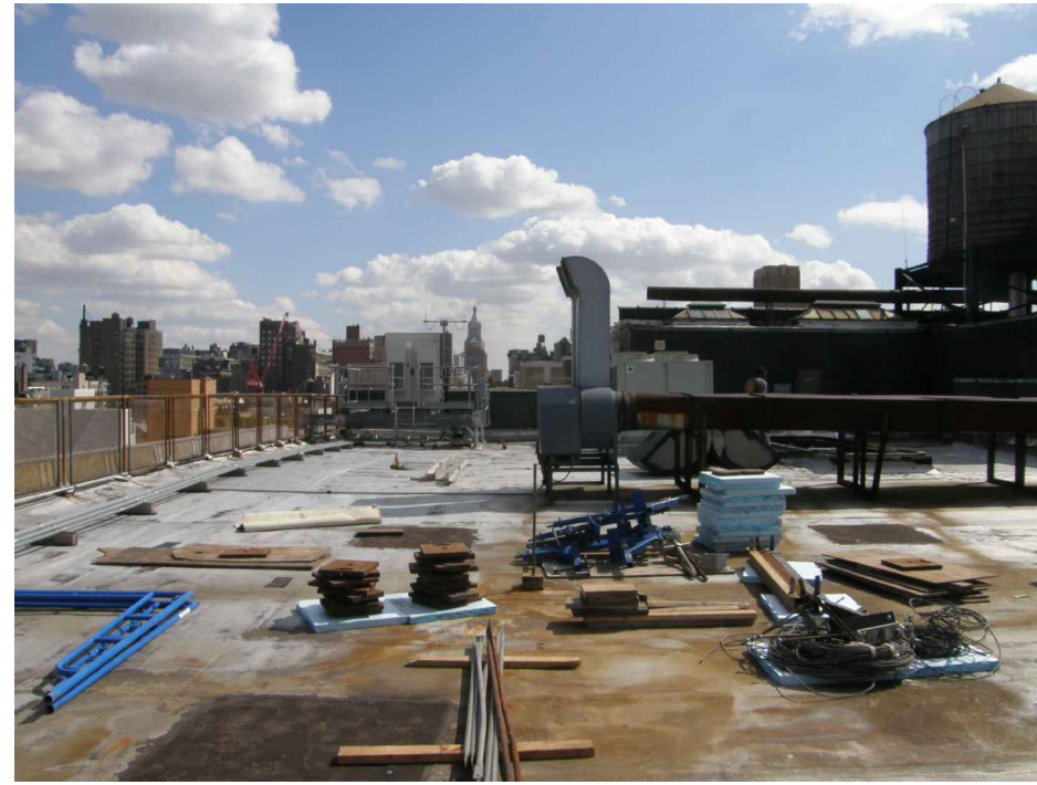
2 EXISTING ROOFTOP EQUIP. EXISTING
