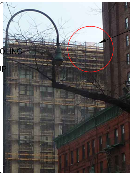
5 DETAIL PHOTO MOCK-UP
