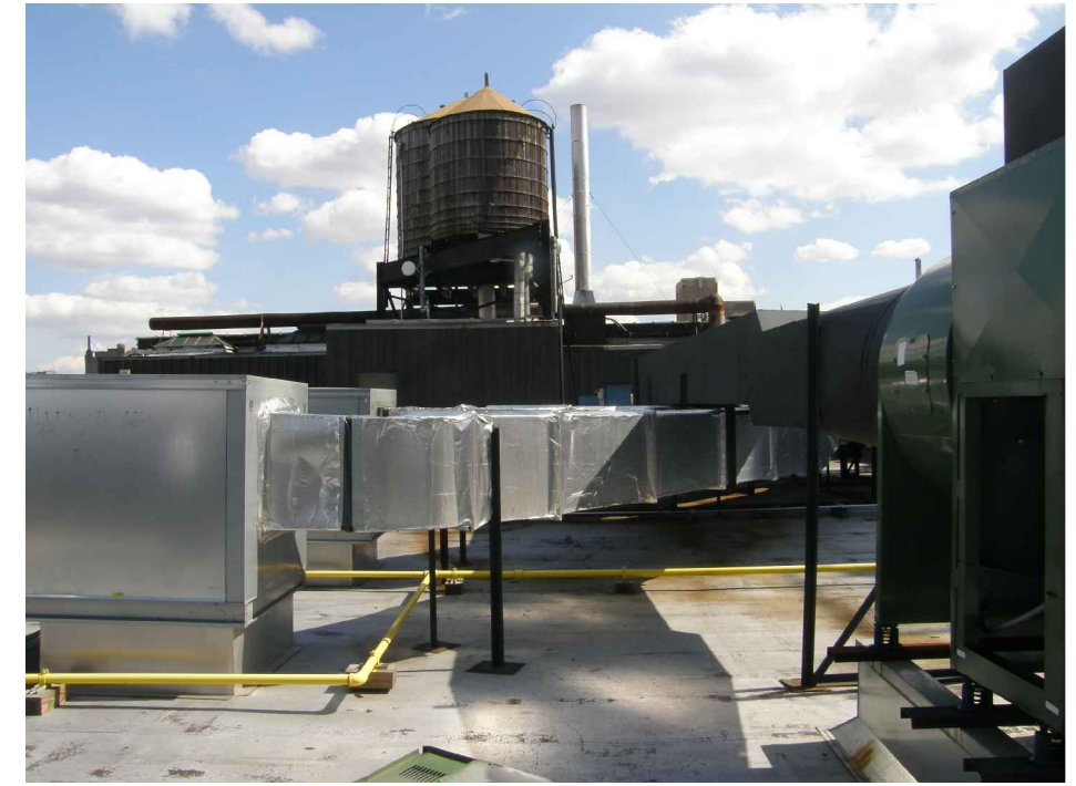
3 EXISTING ROOFTOP EQUIP. EXISTING
