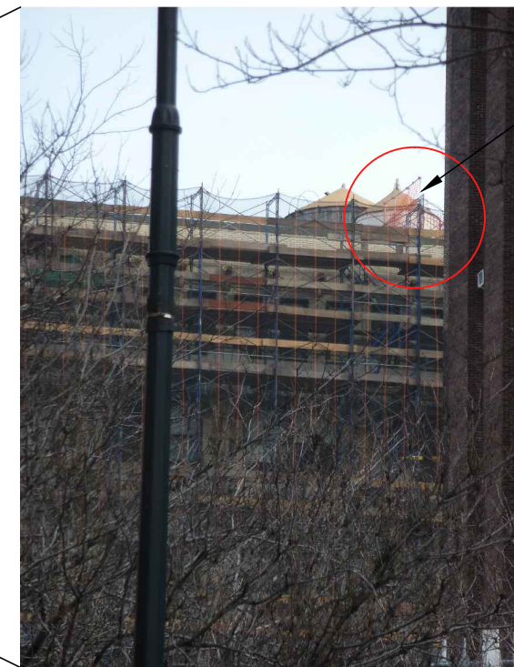
3 DETAIL PHOTO MOCK-UP
