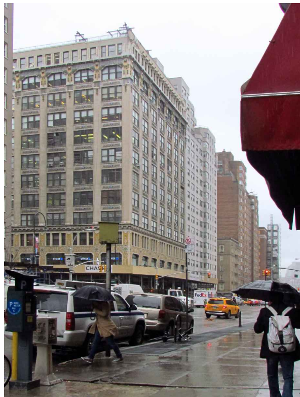
2 VIEW FROM NORTH EXISTING
