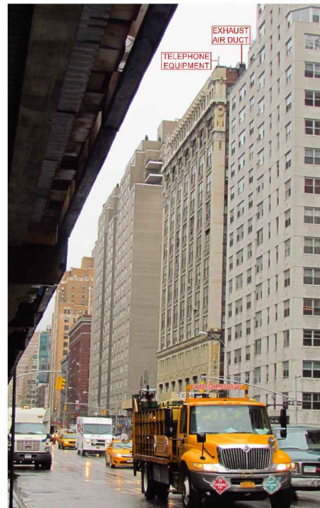
2 VIEW FROM SOUTH EXISTING
