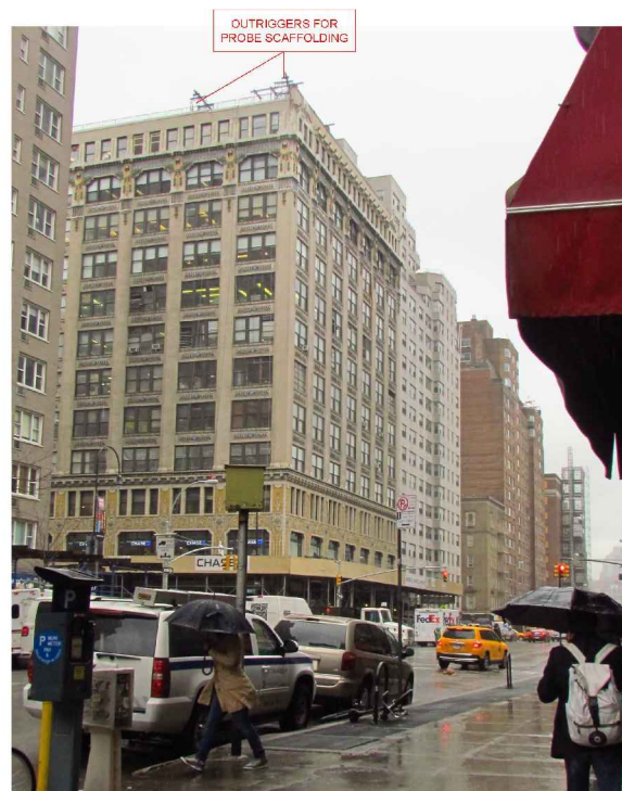
2 VIEW FROM NORTH EXISTING
