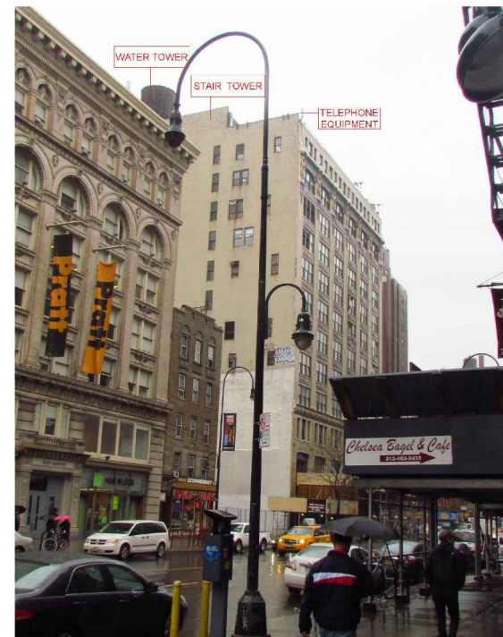
4 VIEW FROM EAST EXISTING
