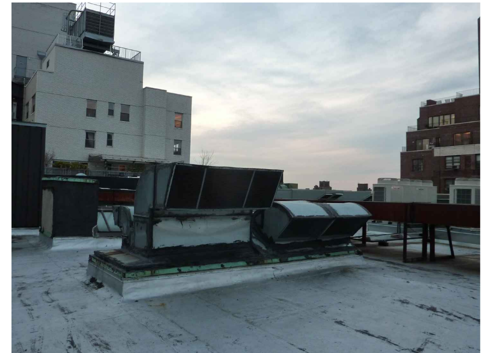
5 EXISTING ROOFTOP EQUIP. EXISTING
