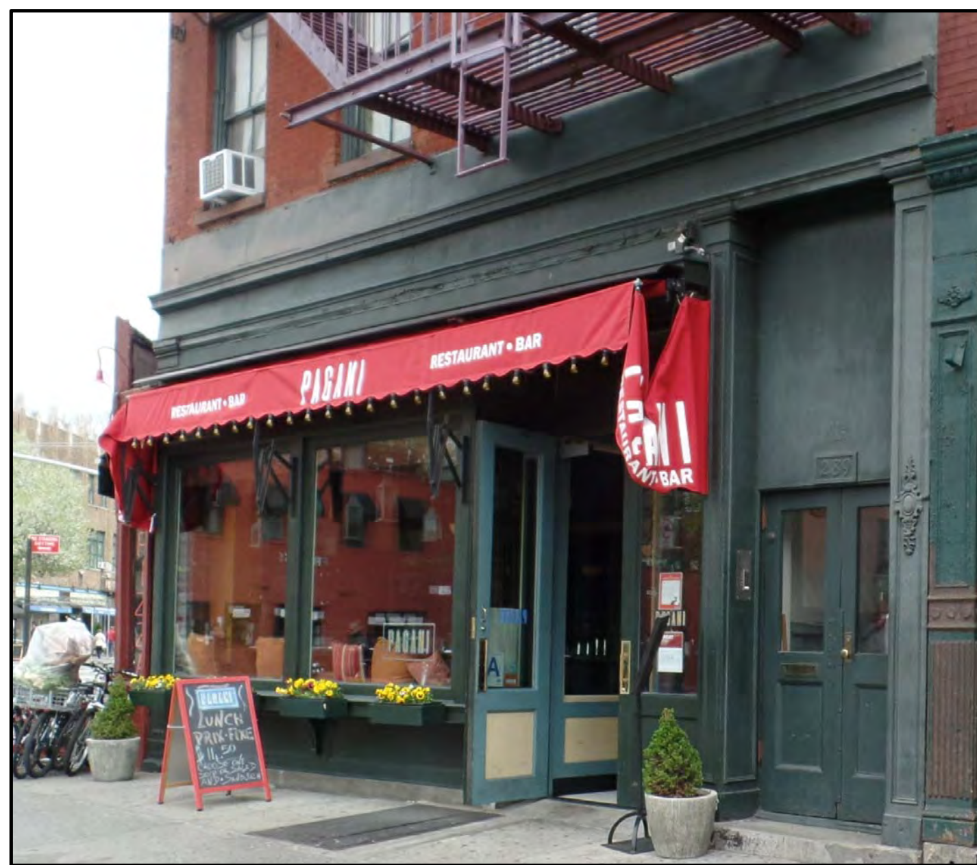
VIEW LOOKING NORTH AT 7TH AVE SOUTH
