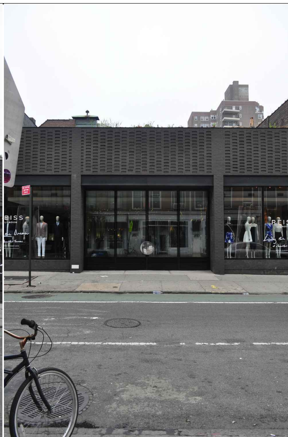
PHOTOGRAPH #2 BLOCK 591 - BLEECKER ST 2 A-402 MAY 18, 2015
