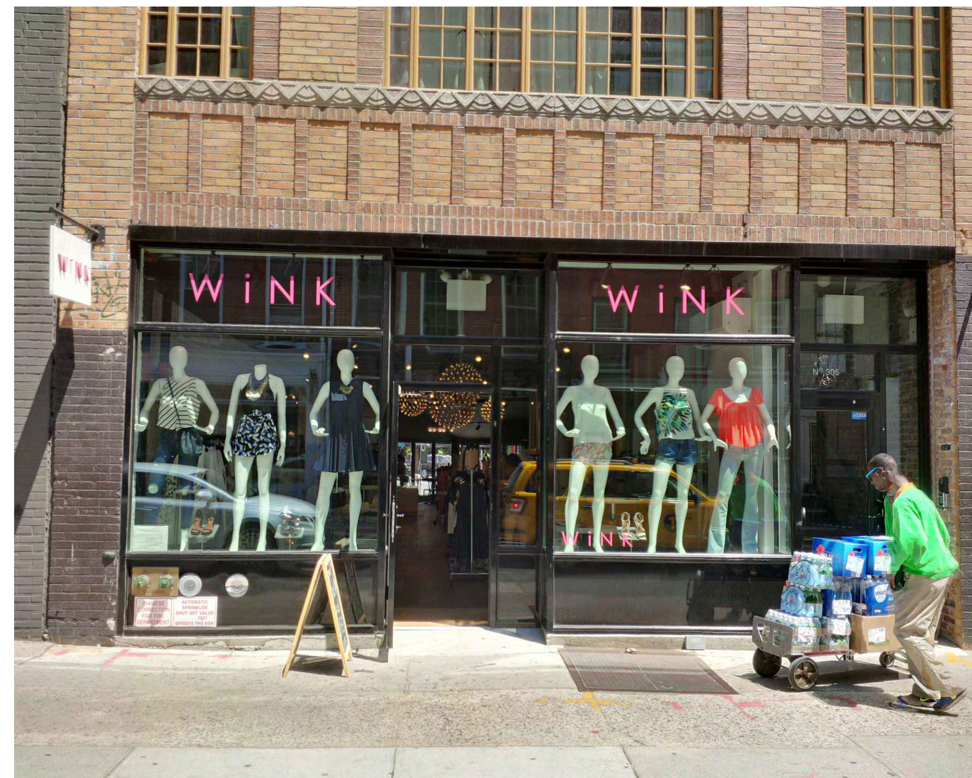
PHOTOGRAPH #3 305 BLEECKER STREET 3 A-403 MAY 14, 2015
