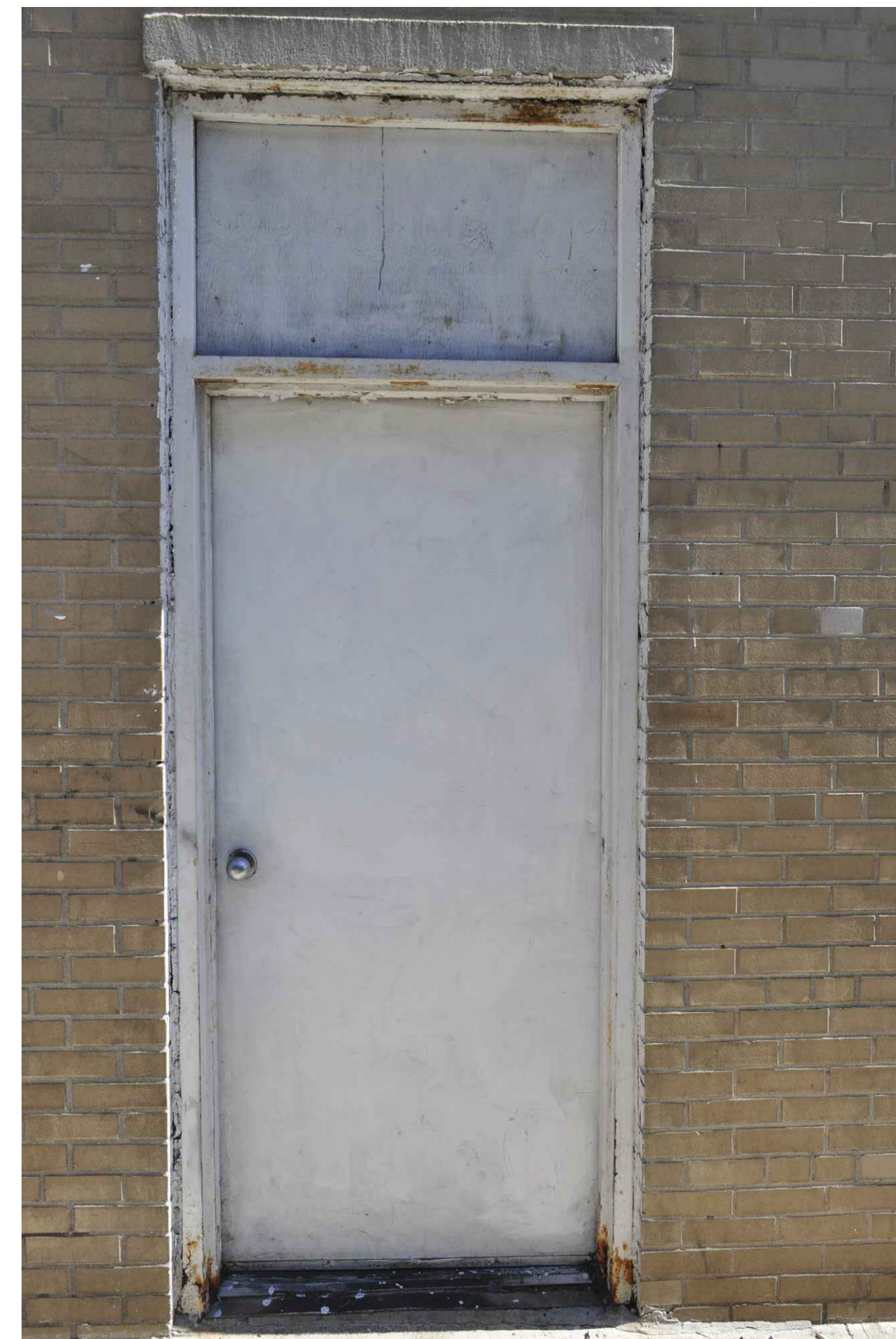
PHOTOGRAPH #4 303 BLEECKER STREET 4 A-400 SEPTEMBER 23, 2014
