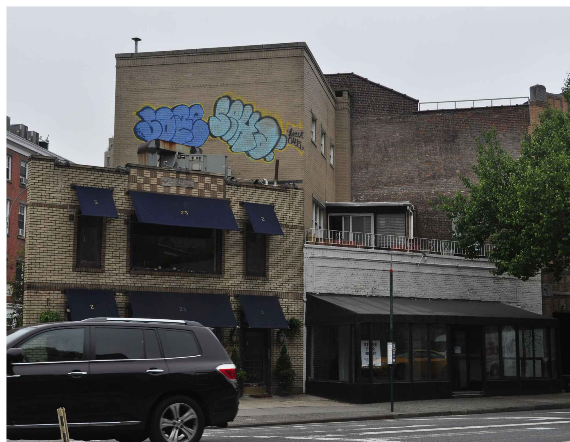
PHOTOGRAPH #2 84-86 7TH AVENUE SOUTH JUNE 18, 2015
