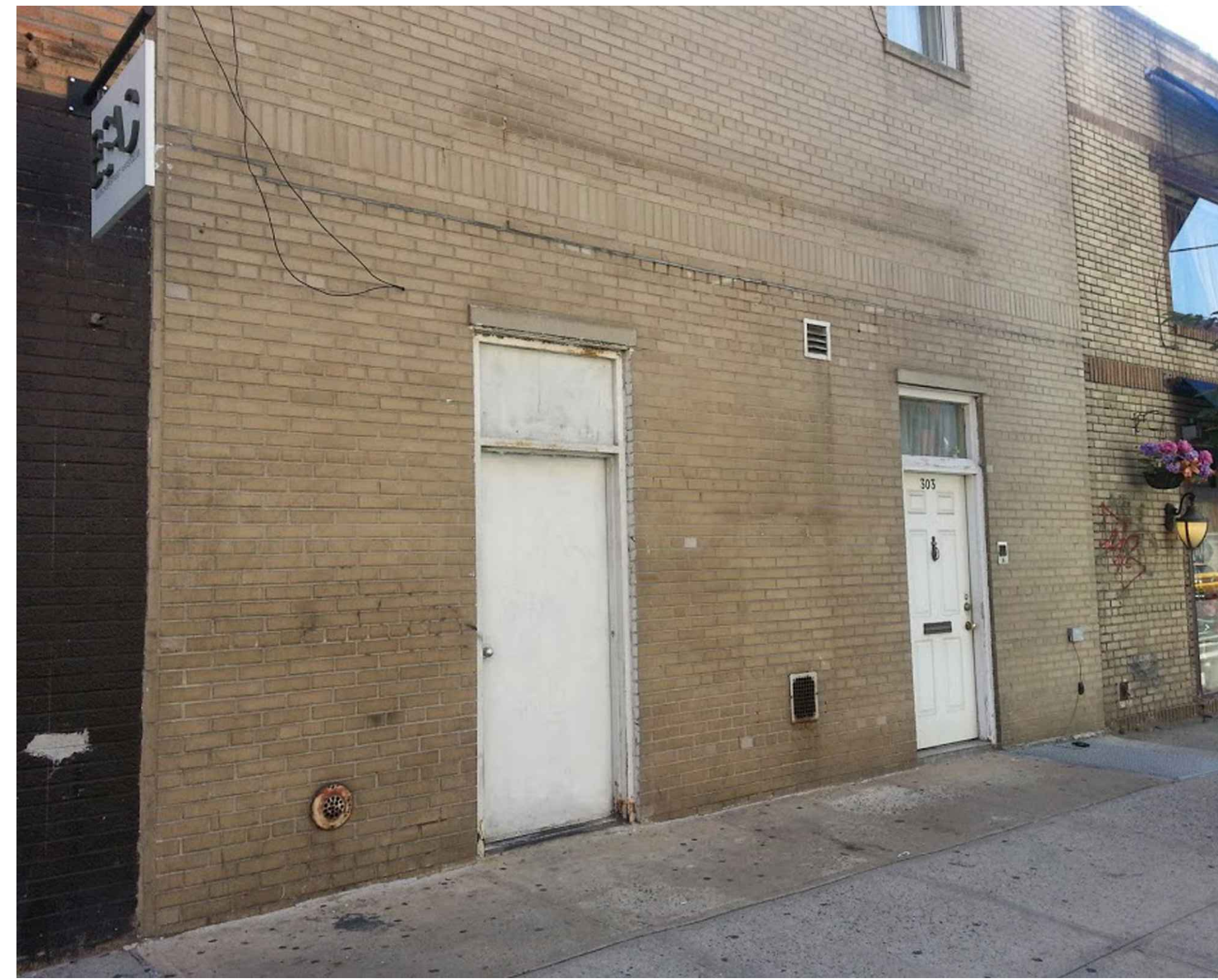
PHOTOGRAPH #1 303 BLEECKER STREET 1 A-400 MAY 30, 2013
