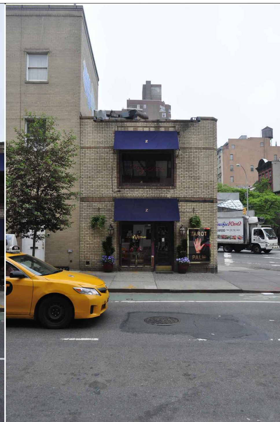
PHOTOGRAPH #6 BLOCK 591 - BLEECKER ST 6 A-402 MAY 18, 2015
