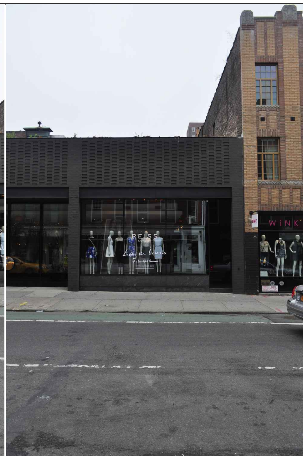
PHOTOGRAPH #3 BLOCK 591 - BLEECKER ST 3 A-402 MAY 18, 2015
