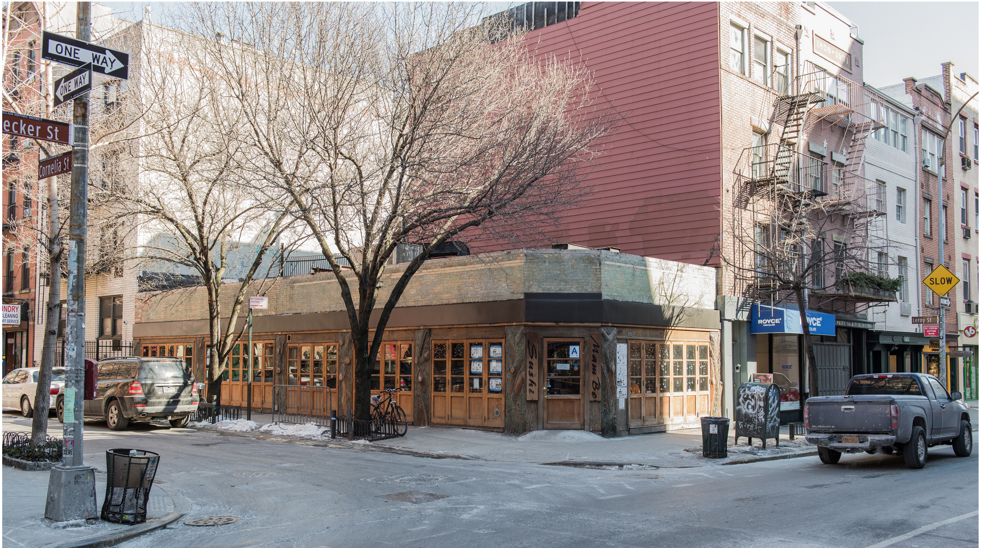
255 BLEECKER STREET — EXISTING BUILDING, STREET APPROACH FROM NORTH SIDE
