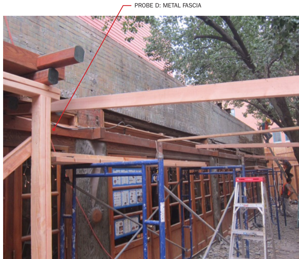
8. PROBE AT WOOD HEADER INFILL, IMAGE FROM PREVIOUS RENOVATION
