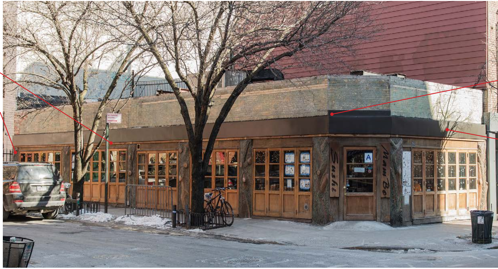
255 BLEECKER STREET FROM NW CORNER
