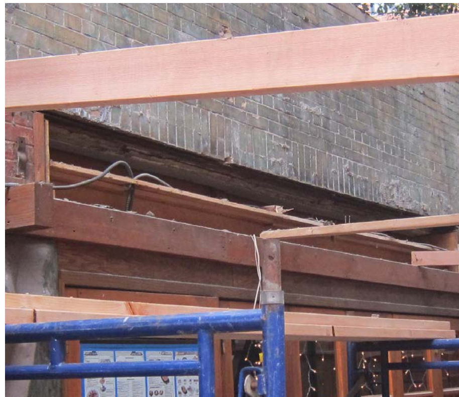
9. PROBE AT WOOD HEADER INFILL, IMAGE FROM PREVIOUS RENOVATION
