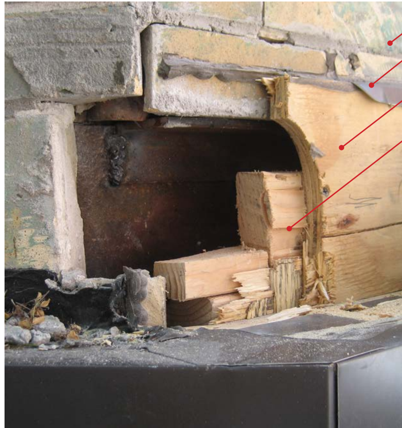
2. PROBE AT NW CORNER DOOR HEADER
