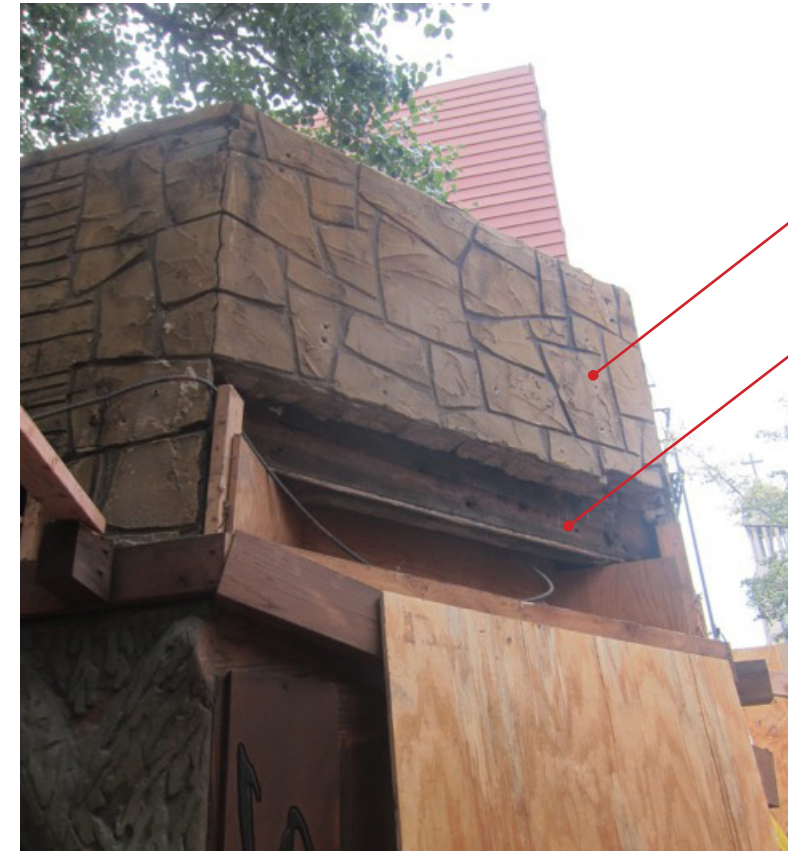
4. PROBE AT NW CORNER DOOR HEADER, IMAGE FROM PREVIOUS RENOVATION
