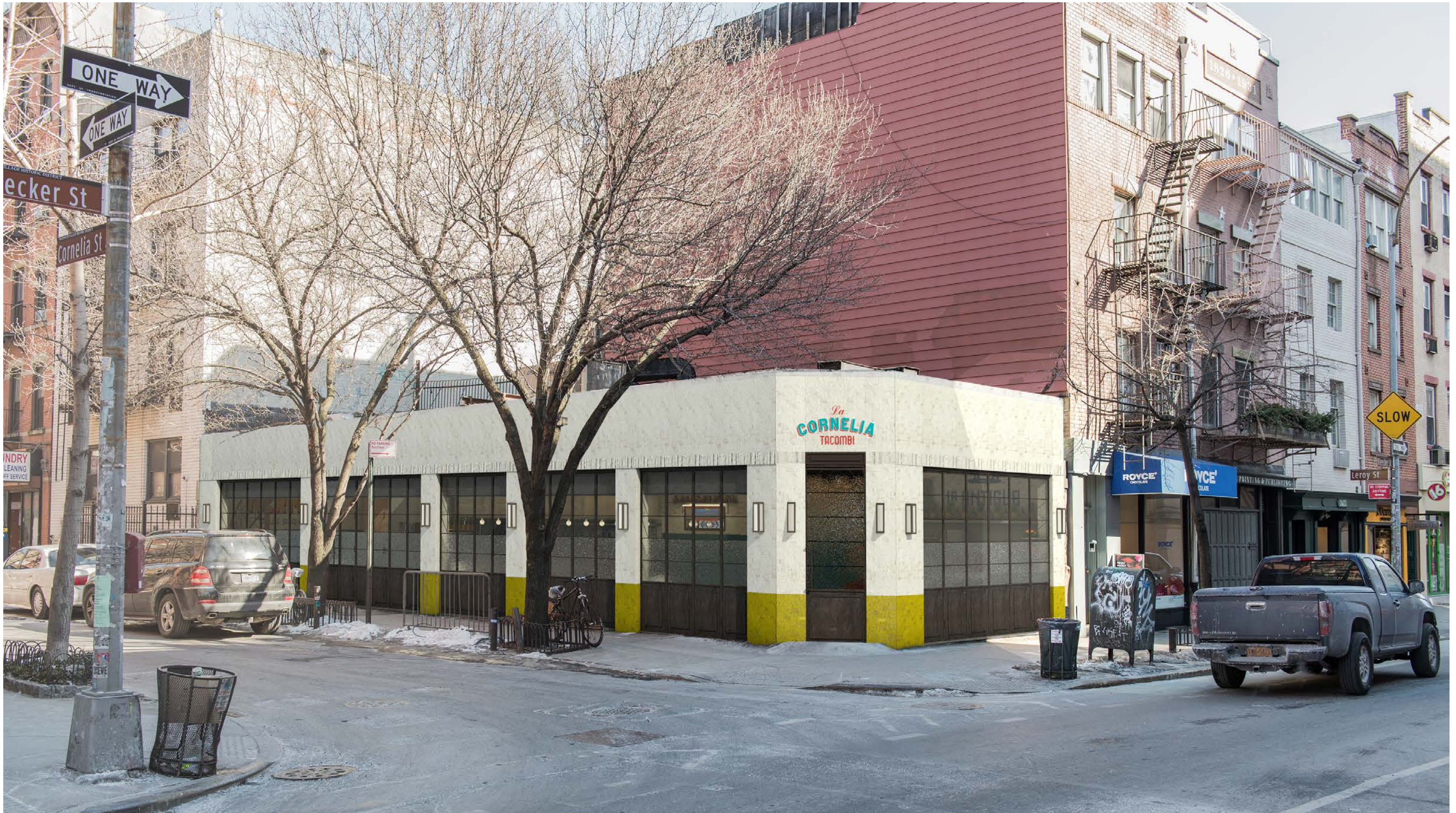
VIEW FROM WEST AT CORNER OF BLEECKER AND CORNELIA STREETS
