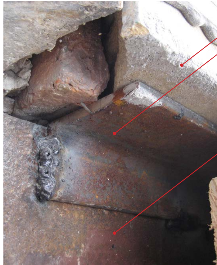
3. PROBE AT NW CORNER DOOR HEADER
