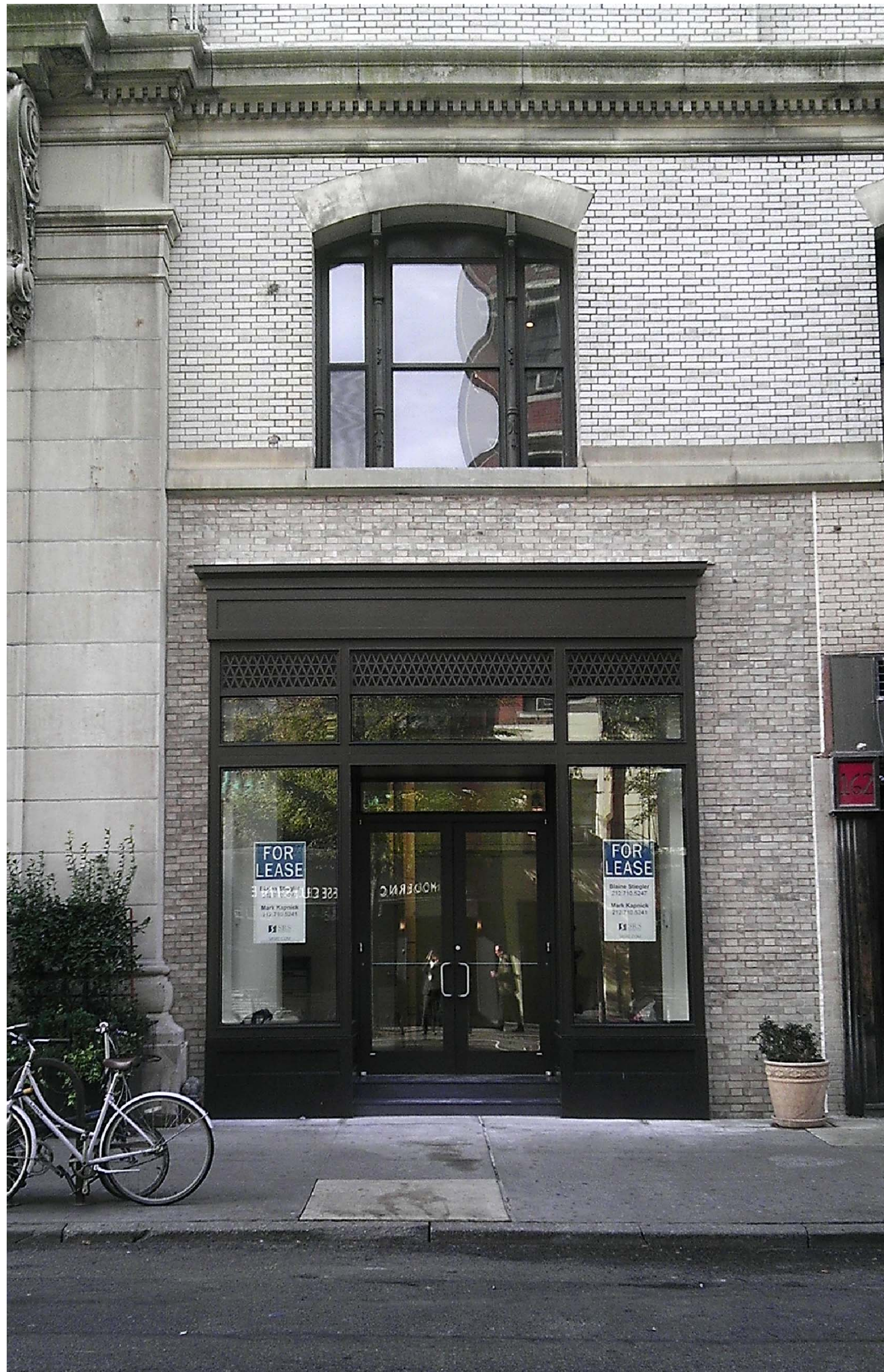
VIEW FROM ACROSS STREET
