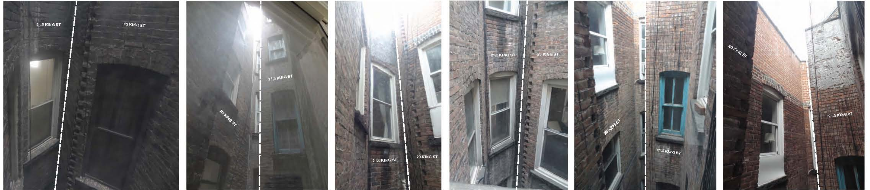
VIEW OF EXISTING CENTER WEST LIGHTWELL FROM 2ND FLOOR TO 5TH FLOOR
