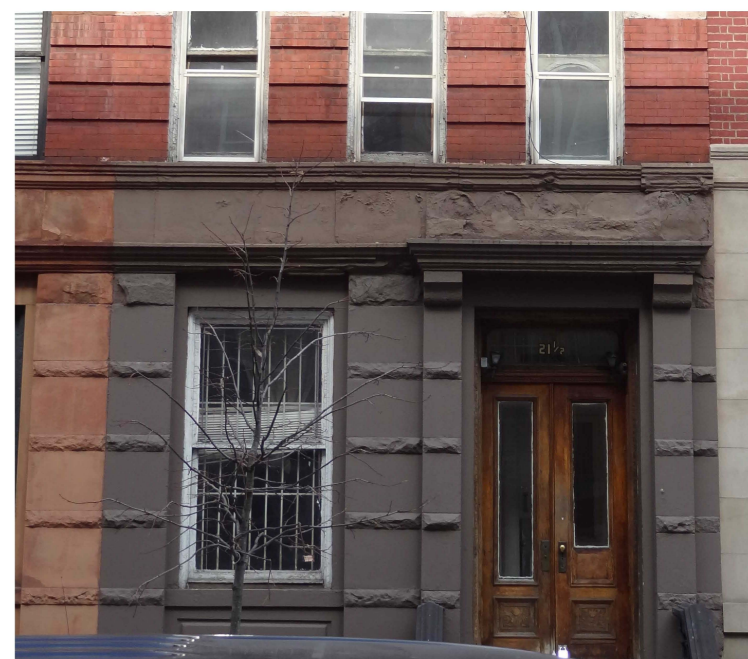
SOUTH FACADE AT 1ST FLOOR - 21.5 KING STREET
