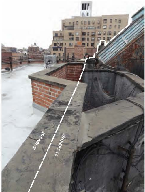
EXISTING CENTER LIGHTWELL ALONG WEST LOT LINE (LOOKING NORTH)
