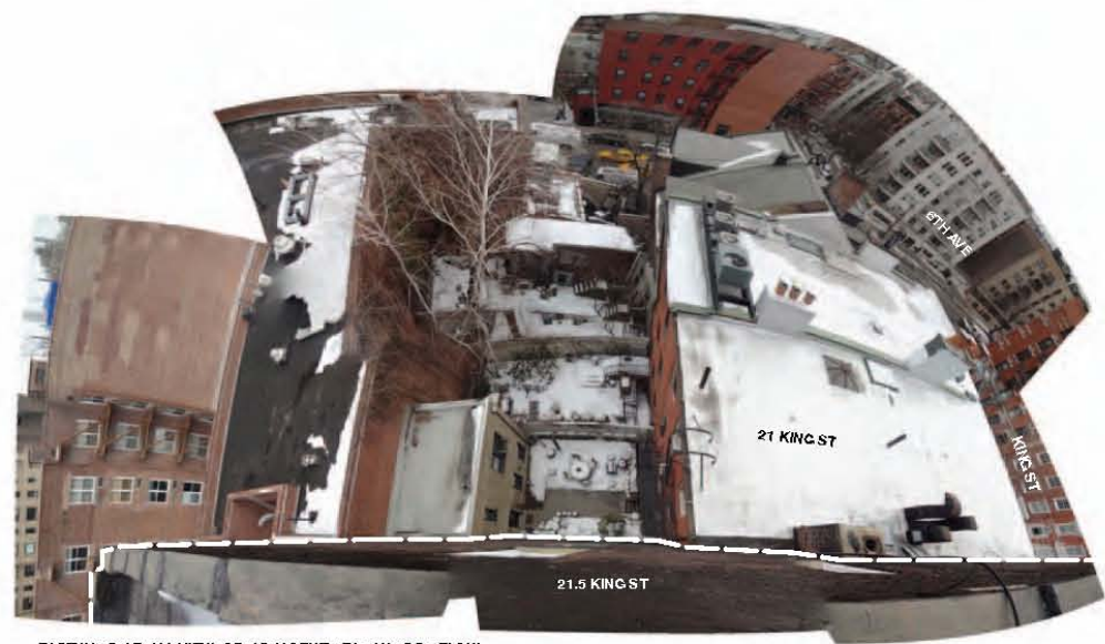
EASTWARD AERIAL VIEW OF ADJACENT REAR YARDS BELOW
