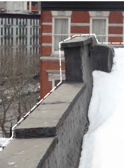
EXISTING SOUTHEASTERN PARAPET CORNER (6TH AVE BEYOND)
