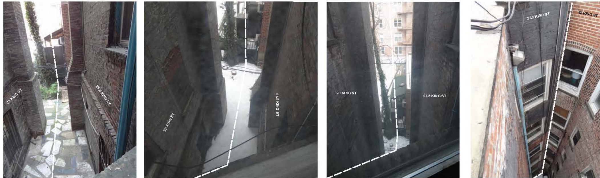
VIEW OF EXISTING NORTH WEST LIGHTWELL FROM 1ST FLR TO ROOF
