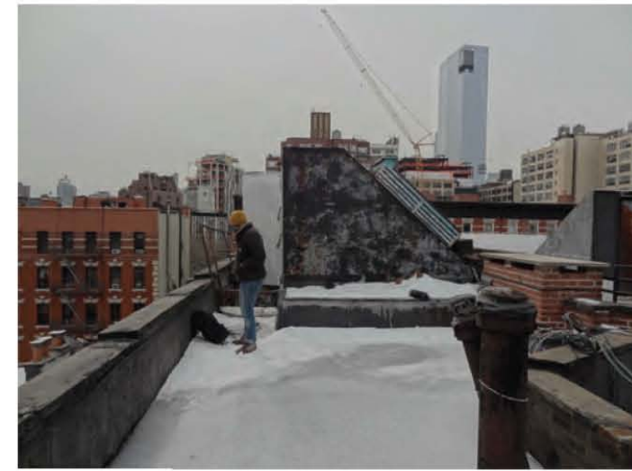
EXISTING ROOF (LOOKING SOUTH)
