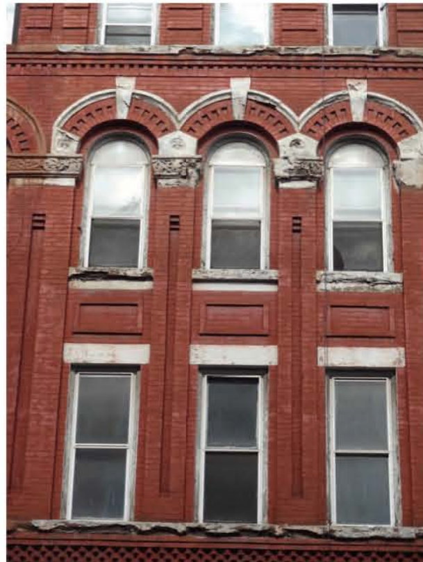
3RD & 4TH FLOOR WINDOWS AT SOUTH FACADE - PLEXI-VINYL STORM WINDOW APPLIED OVER EXISTING WOOD WINDOW - HEAVILY SPALLED & PAINTED BROWNSTONE MOULDINGS & DETAILS
