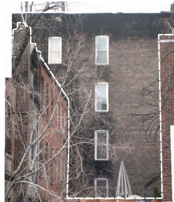
6TH AVENUE DETAIL VIEW OF EAST WALL SEEN THROUGH REAR YARD / INTERIOR OF BLOCK
