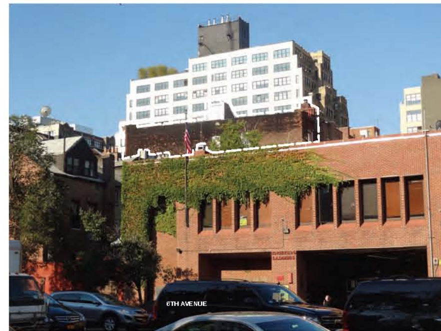
SOUTH WESTERN VIEW ALONG 6TH AVE SEEN FROM OPPOSITE SIDEWALK
