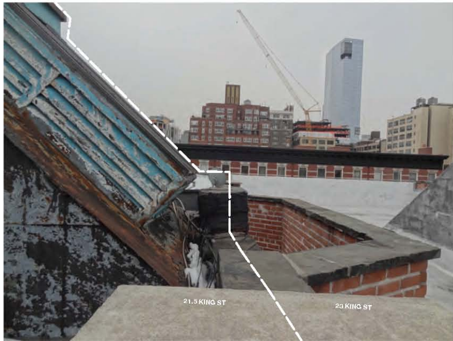
EXISTING BULKHEAD & LIGHT WELL ALONG WEST LOT LINE (LOOKING SOUTH)
