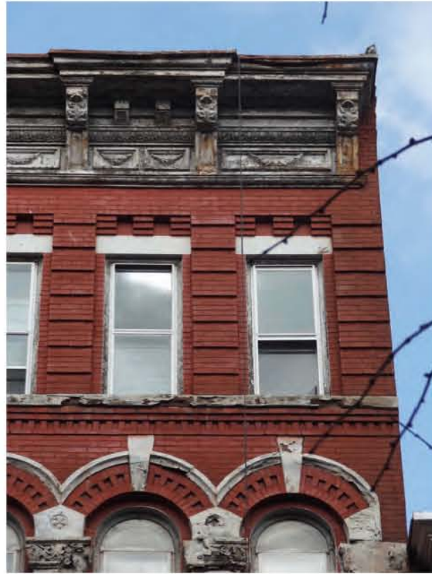
CORNICE, 4TH & 5TH FLOOR WINDOWS AT SOUTH FACADE - PLEXI-VINYL STORM WINDOW APPLIED OVER EXISTING WOOD WINDOW - HEAVILY SPALLED & PAINTED BROWNSTONE MOULDINGS & DETAILS - RUST DAMAGE AT PORTIONS OF CAST IRON CORNICE
