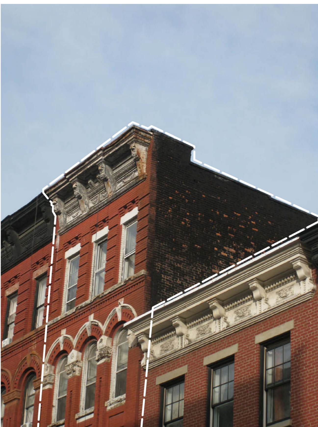
SE CORNER DETAIL VIEW OF 21.5 KING STREET FROM OPPOSITE STREET CORNER
