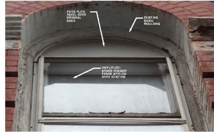
INTERIOR & EXTERIOR DETAIL VIEWS OF TYPICAL PLEXI-VINYL STORM WINDOW AT SOUTH FACADE. PLEXI PANEL OVER EXISTING DOUBLE HUNG WINDOWS W/ ARCHED GLASS LIGHT IN UPPER SASH.
