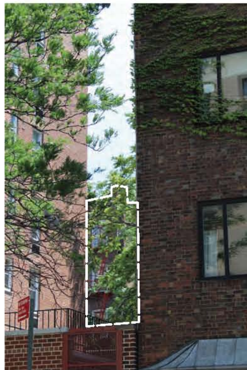
WEST HOUSTON ST. VIEW OF REAR YARD (NORTH) FACADE THROUGH INTERIOR BLOCK
