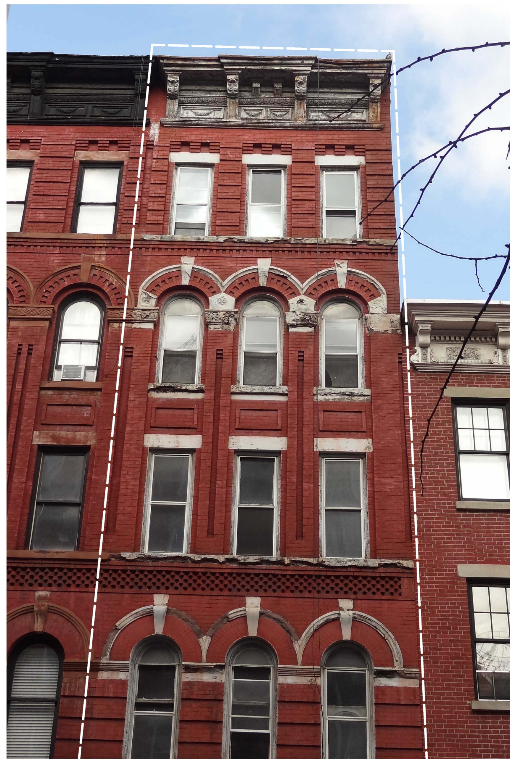
SOUTH FACADE 2ND THROUGH 5TH FLRS - 21.5 KING STREET
