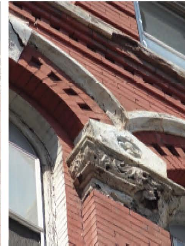
DETAIL OF 4TH FLOOR WINDOW AT SOUTH FACADE - PLEXI-VINYL STORM WINDOW APPLIED OVER EXISTING WOOD WINDOWS - HEAVILY SPALLED & PAINTED BROWNSTONE MOULDINGS & DETAILS
