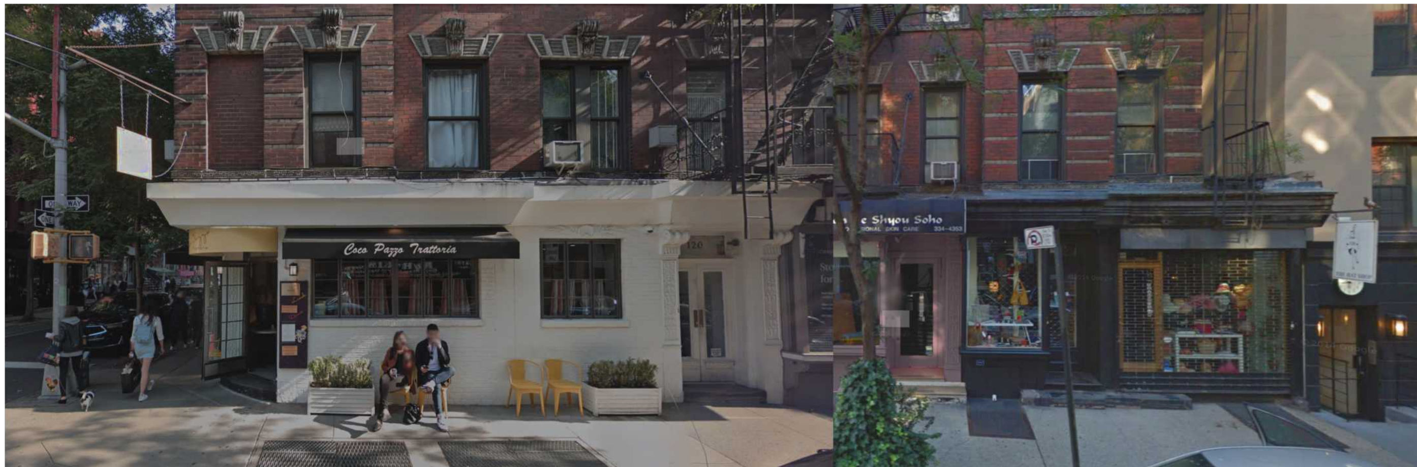
THOMPSON STREET STOREFRONT ELEVATION PHOTO
