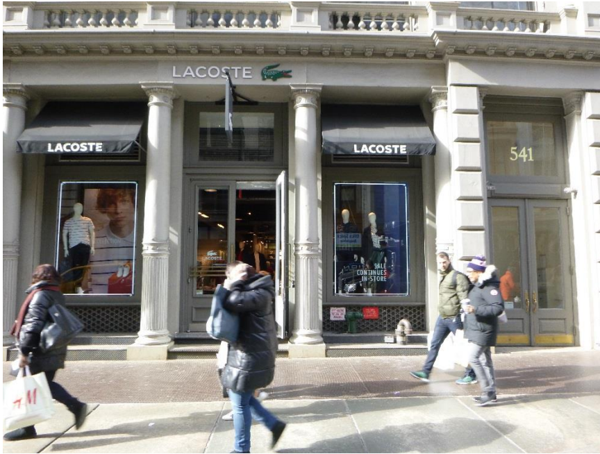
STREET VIEW: SIDEWALK VAULT – AFTER REPAIRS TO DIAMOND PLATE
