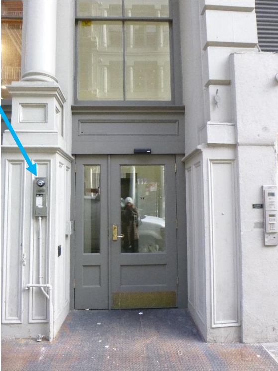
112 MERCER STREET ENTRANCE INTERCOM AS CURRENTLY INSTALLED
