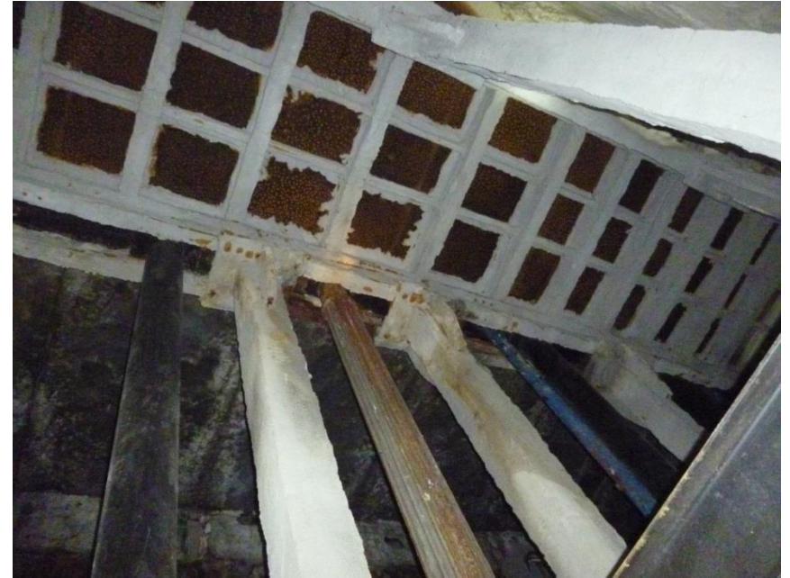
VAULT VIEW: SIDEWALK VAULT AFTER REPAIRS
