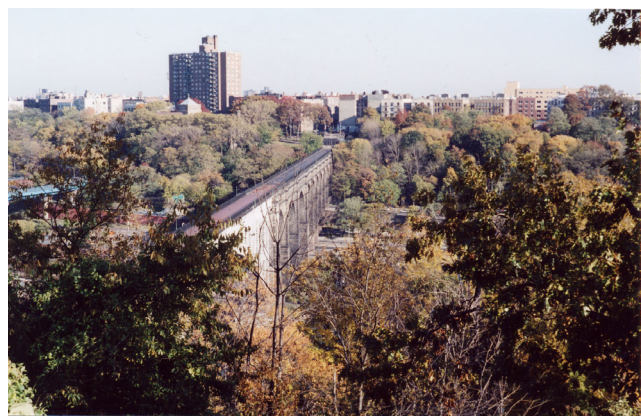
High Bridge is the oldest Harlem River span still in existence.
