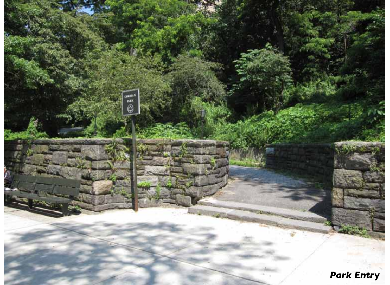
Retaining Wall; Setback From Street Wall
