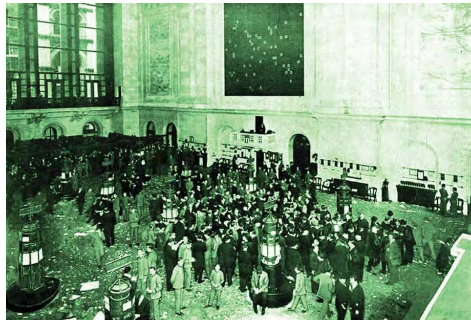
New York Stock Exchange Floor - 1908 The first central location of the Exchange was a room, rented in 1817 for $200 a month, located at 40 Wall Street.
