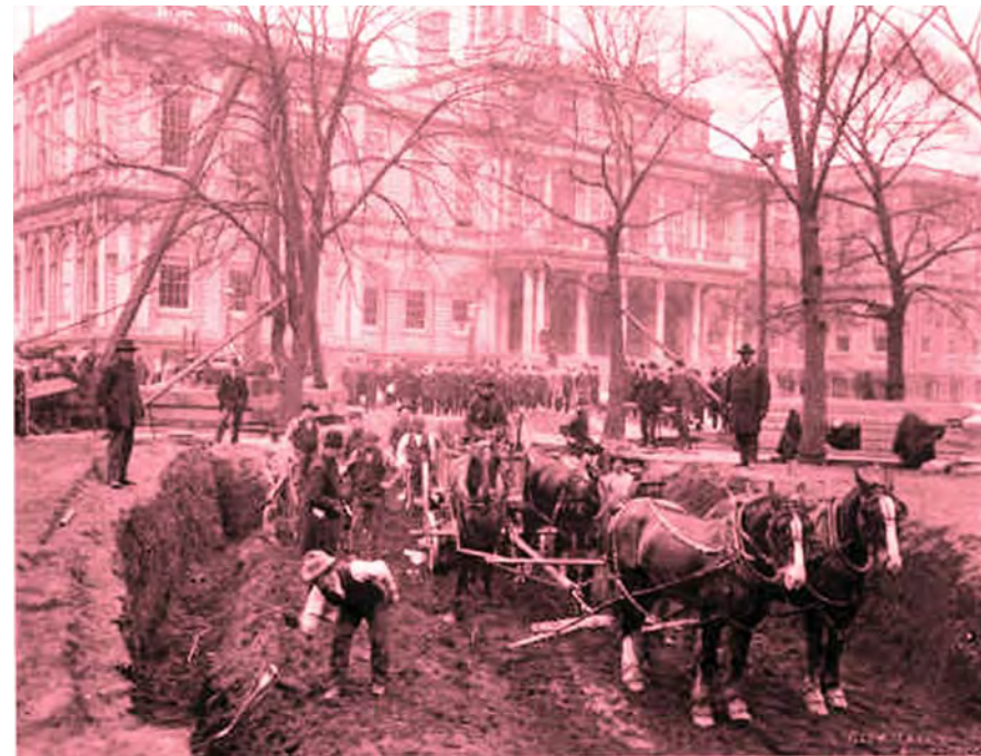
City Hall Park during subway construction - 1901 In 1901, subway construction methods involved tearing up streets to dig the tunnel below, and then rebuilding the street above.
