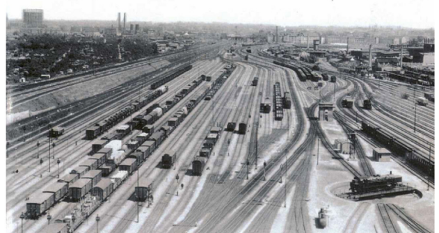
Photo of the switchyard in 1935 (taken from the watertower) by Carl Bellingrodt
