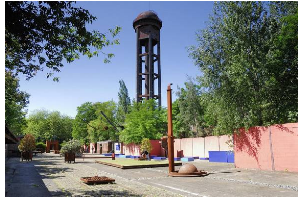
Photo of the historic water tower and view from the Italian garden ("Giardino Segreto")
