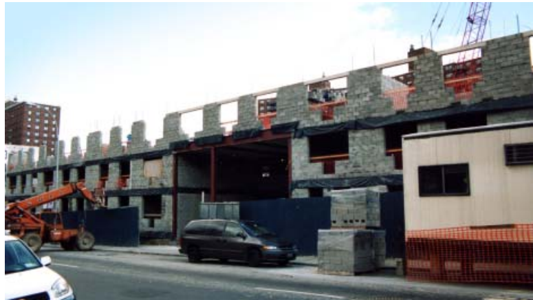
A LAMP project under construction at 1240 Washington Avenue in the Bronx
