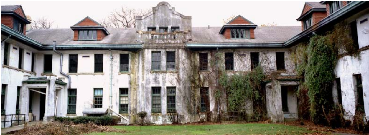
The rehabilitation of the former nurse's residence located on the Sea View Hospital Rehabilitation Center and Home campus in the Willowbrook section of Staten Island will create approximately 100 units of senior citizen housing.
