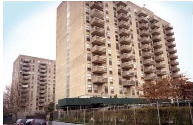
North Shore Plaza in Staten Island is the first Mitchell-Lama development to receive $1.5 million to repair 535 units.
