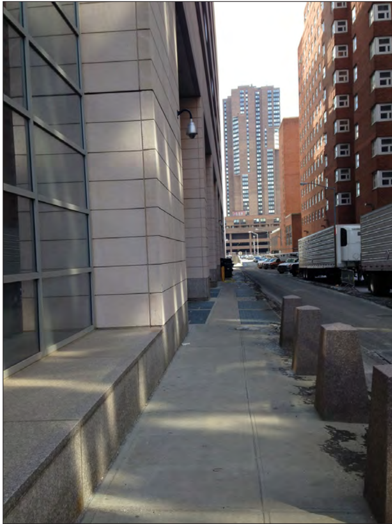
. View of hospital building, facing east 3
