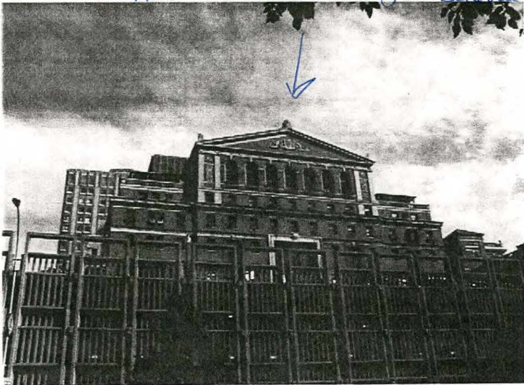
23. View of the western facade of the Parking Garage with the upper facade of the administration building above and the inpatient hospital building seen behind. Taken from First Avenue and East 28 th Street.
