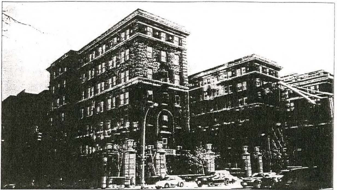
Psychiatric Building, looking southeast from First Avenue and East 30th Street 1
