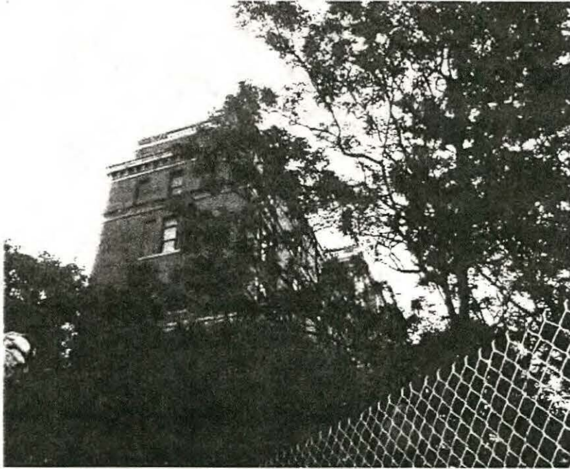
7. View of the western facade's corner from the hospital parking lot
