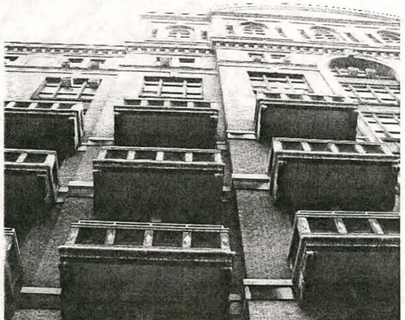
9. View of the southern facade from the Ambulance Garage
