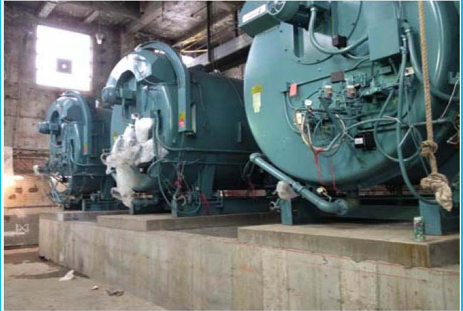
Three new 500 HP boilers on new supports.
