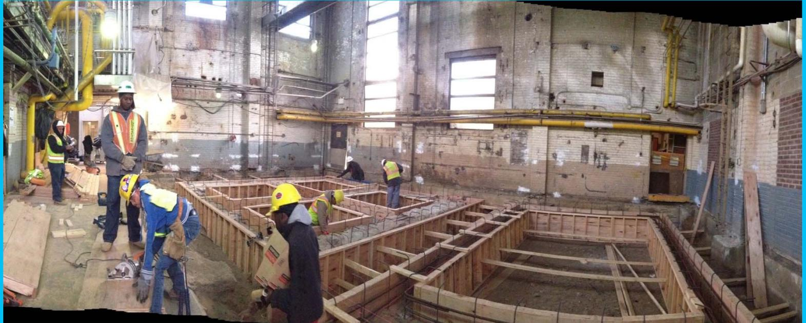
Structural repairs incorporating resiliency design of boiler room floor after damage from Hurricane Sandy .
