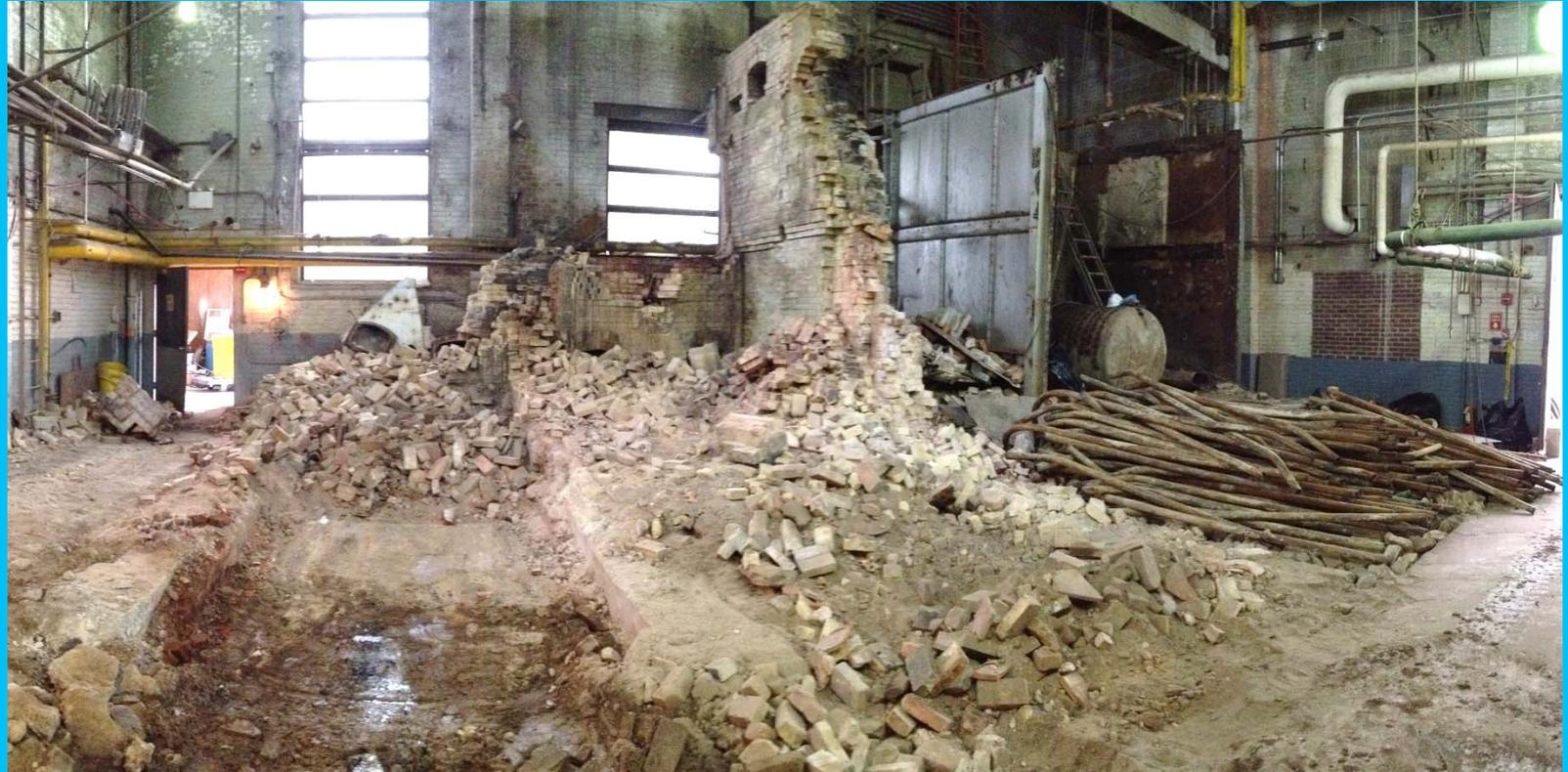
Post Sandy demolition of boilers installed in 1930's and 1950's
