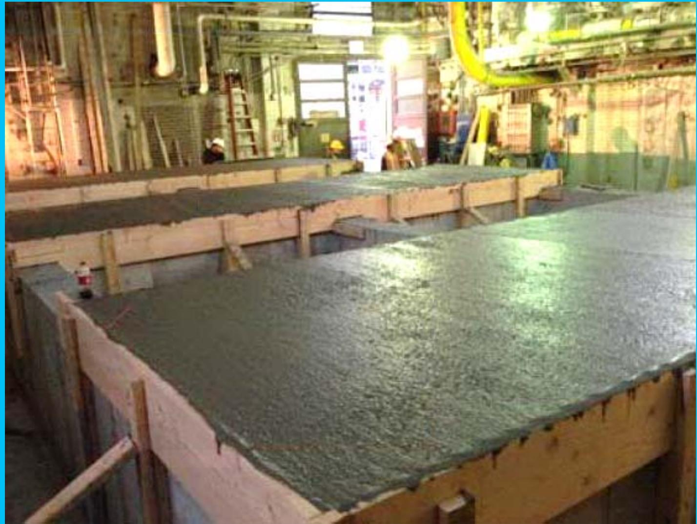
New boiler supports are elevated above FEMA 100-yr flood line
