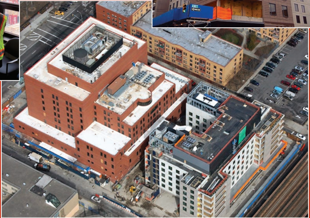
Right: Top view, showing the existing hospital building (red brick structure on left), which is being renovated, and the new construction (gray building on right) as of February 19, 2013.
