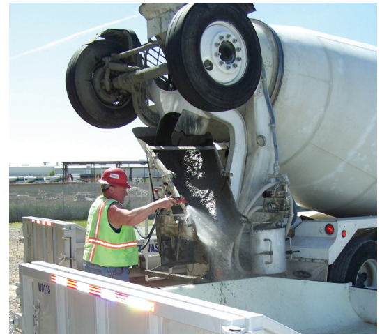
HT 13: Concrete washout water has a pH comparable to Drano® Clog Remover.
