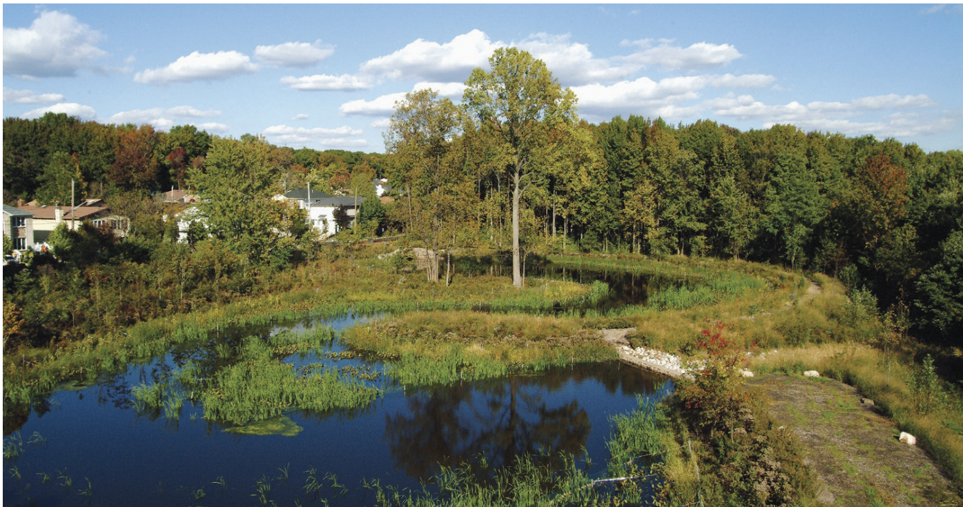
SW 5: The Staten Island “Bluebelt.” Stormwater can be controlled with properly engineered natural systems.
