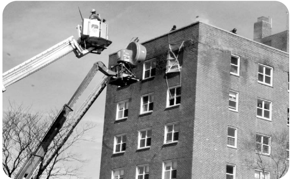
A fire curtain is used by firefighters to block the wind (generated by a large fan) from a raging apartment fire on Governors Island during a weeklong study of wind-driven high-rise fires.
