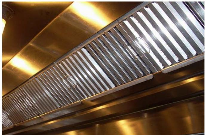
All baffle filters must be installed with the baffles running vertically so the grease can drain downward and out of the weep holes. Notice that all baffle filters should have weep holes in the bottom of the filter so grease can
