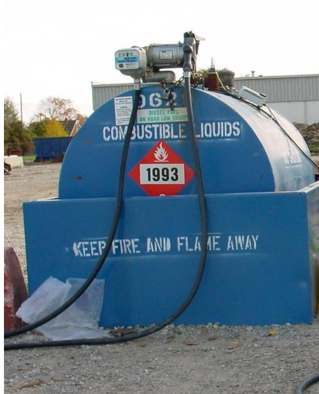
Example of a temporary tank with top openings.
