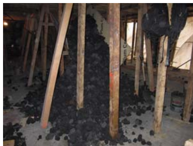
Unsafe (in orderly) stored coke
