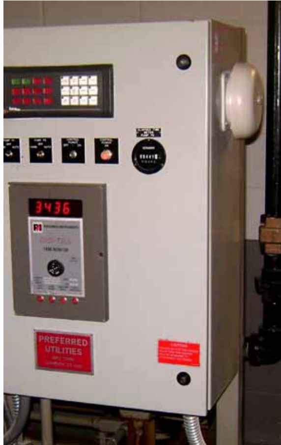
Working indicator with audible alarm attached; DIAGRAM
