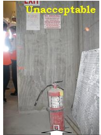
Improper floor placement of Fire Extinguisher.
