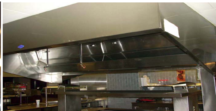
Type I hood Water Wash has cartridge filters & self-cleaning Feature
