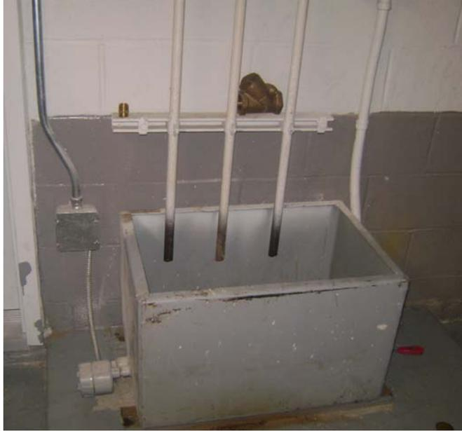
**“Overflow catch Basin” or Tank with attached leak detection alarm**
