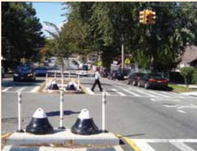
Refuge islands and a landscaped median provide safer crossings and improve the streetscape along Allerton Avenue.
