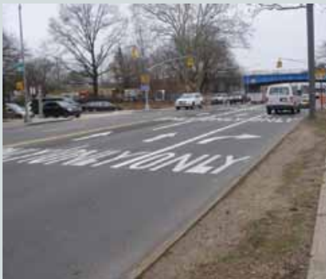
An additional southbound lane designated for westbound Belt Parkway vehicles was added on Bay Parkway to improve traffic operations.
