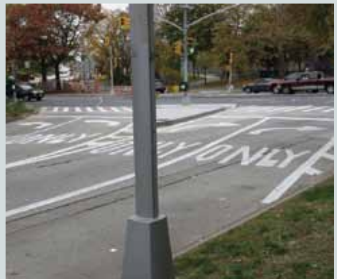
The Belt Parkway westbound exit ramp at Bay Parkway was reconfigured to increase capacity for vehicles exiting the parkway.
