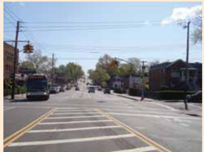
Traffic calming measures applied on Allerton Avenue included the narrowing of the roadway from two lanes in each direction to one and the addition of painted center medians.
