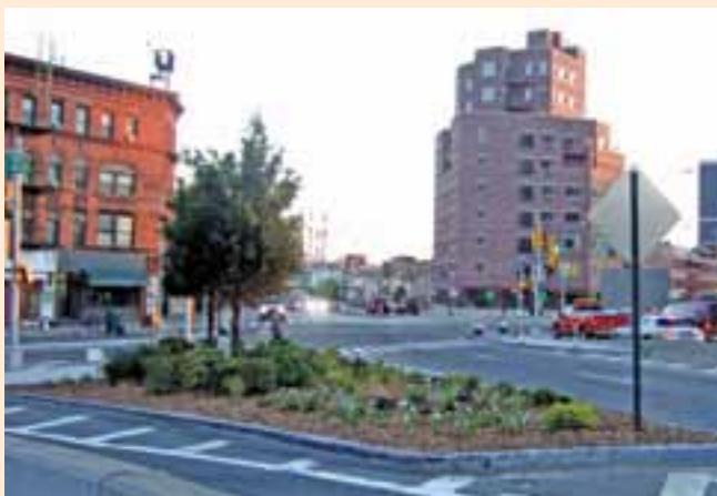
An expanded, landscaped refuge island/median was added at the southwest corner of Jackson Avenue and 11th Street to improve safety for motorists and pedestrians and to enhance the streetscape.
