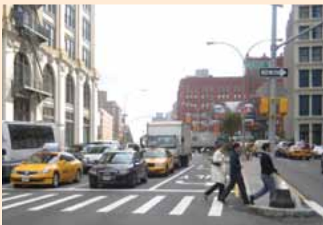
Typical safety improvements along Houston Street included the installation of pedestrian refuge islands, bell bollards, pedestrian ramps, and left-turn bays.
