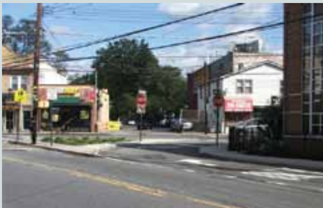
A channelized right-turn lane was constructed at Nelson Avenue for eastbound Amboy Road traffic to help calm traffic.
