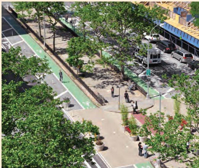
A bird's eye view of the project showing the new bicycle lane, buffer space and a pedestrian plaza created by connecting the malls.
