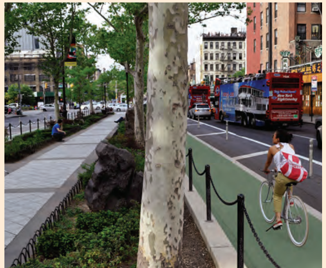
Safety for cyclists was improved by moving the bike lane next to the mall and providing a nine-foot buffer between the bike lane and vehicle travel lanes.
