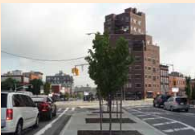
Vehicles at the foot of the Pulaski Bridge can only turn right from the designated right-turn lanes.
