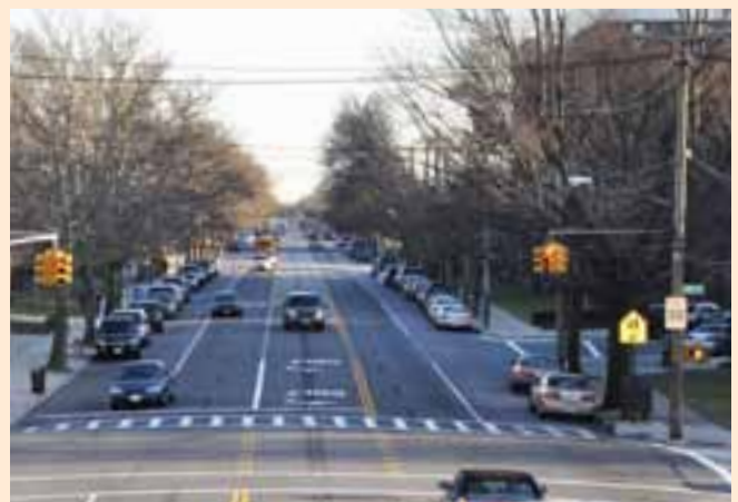
Traffic calming and safety measures applied on Gerritsen Avenue included the narrowing of the roadway from two lanes in each direction to one and the addition of painted center medians and left-turn bays.
