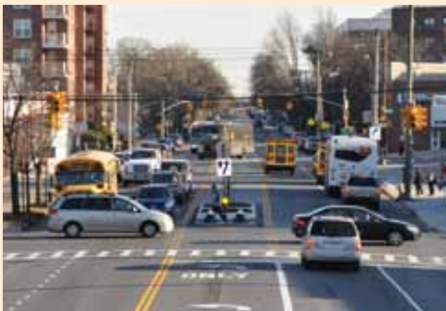
A pedestrian refuge island was installed in the south crosswalk at the intersection of Gerritsen Avenue and Avenue U to improve safety for pedestrians.
