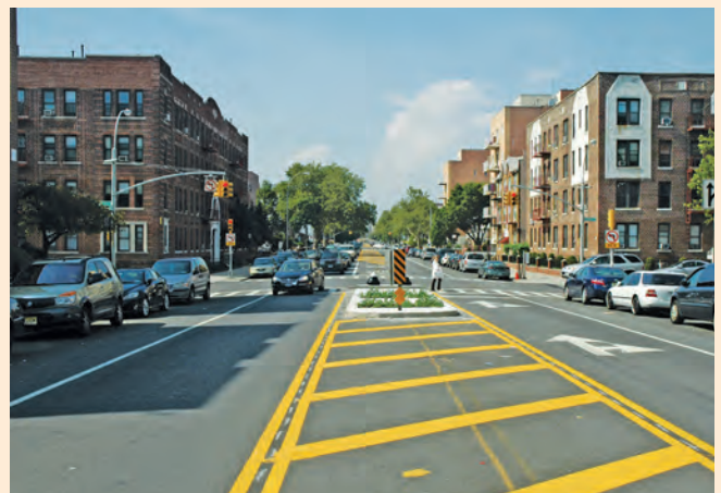
Traffic calming measures applied on West 6th Street included the narrowing of the roadway from two lanes in each direction to one and the addition of painted center medians.
