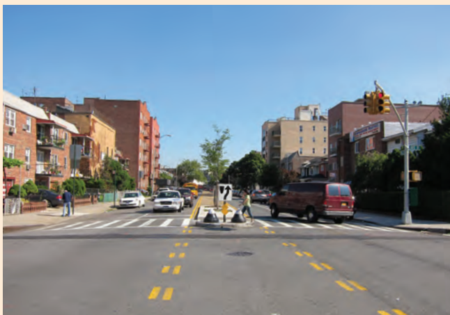
A refuge island, high visibility crosswalk markings and landscaping in the north crosswalk of West 6th Street at Avenue O provides a safer crossing and improves the streetscape.
