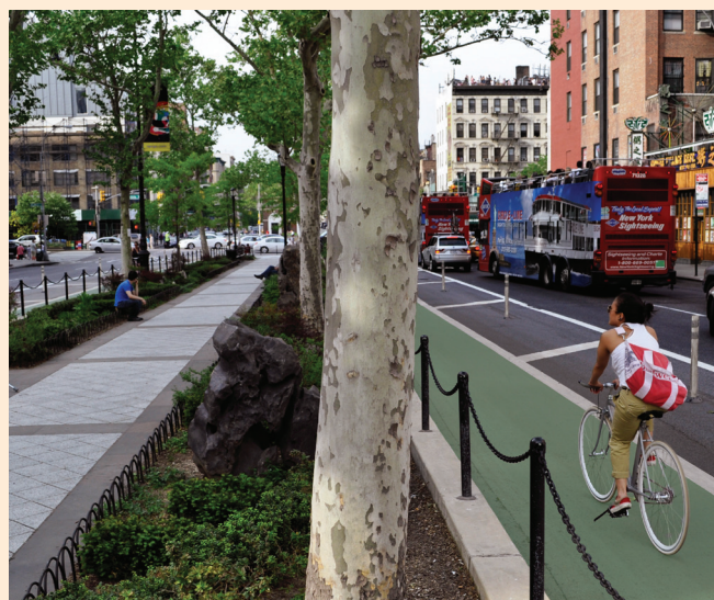
Safety for cyclists was improved by moving the bike lane next to the mall and providing a nine-foot buffer between the bike lane and vehicle travel lanes.
