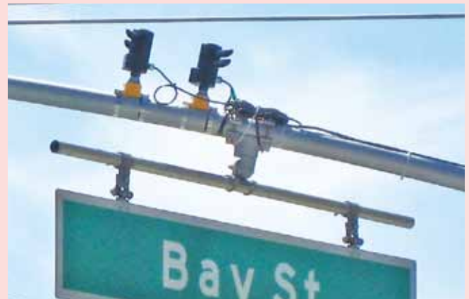
Optical detectors mounted on the traffic signal mast arms at 14 intersections along the study area receive requests from approaching buses.
