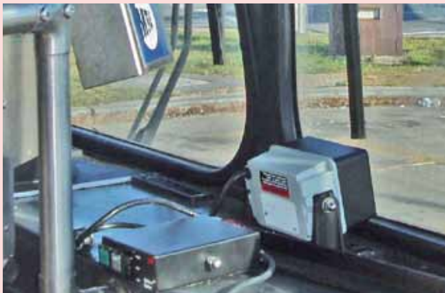
TSP bus emitters were installed in 300 NYCT buses that serve the ferry terminal.
