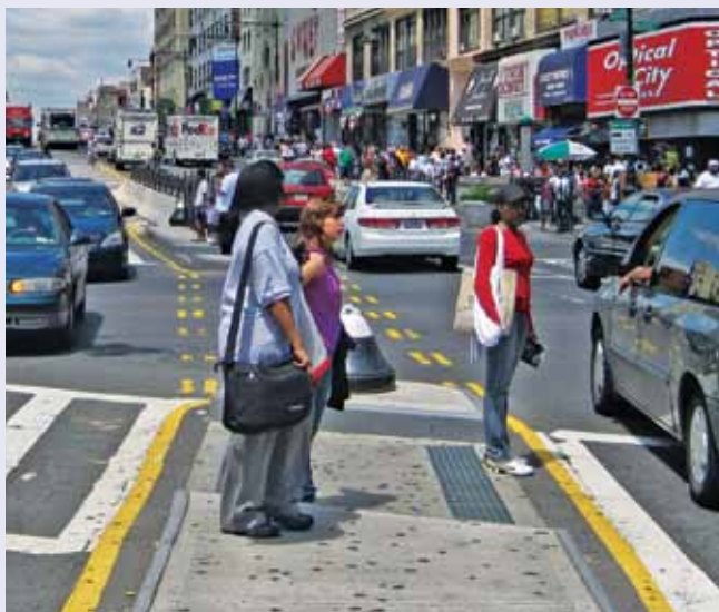
Construction of two new pedestrian refuge islands on E. 149 th Street, reduced a 60 foot crosswalk into two 25 foot sections.
