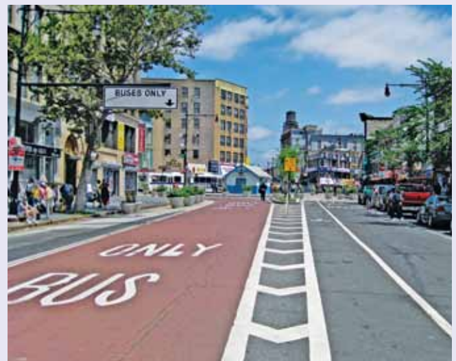
Willis Avenue, north of E. 147 th Street features a dedicated bus lane painted red, a new bike lane and one vehicle travel lane that is diverted right at E. 148 th Street. This allows Willis Avenue to become a plaza.
