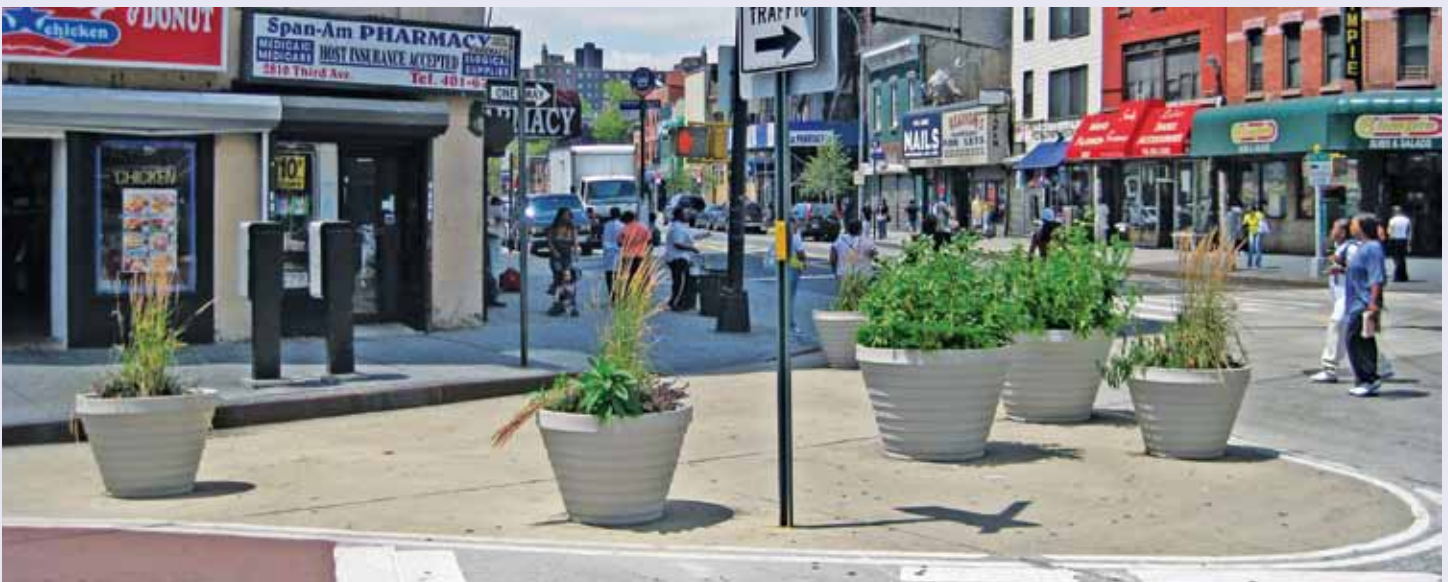
Curb extensions that were installed at four locations helped reduce crossing distances by up to 20 feet.
