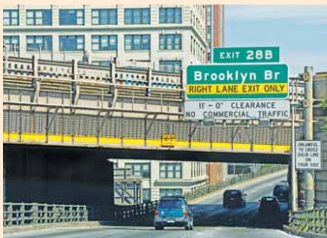
No bridge strikes have been reported at this location since the treatment was installed on the Brooklyn Bridge overpass.
