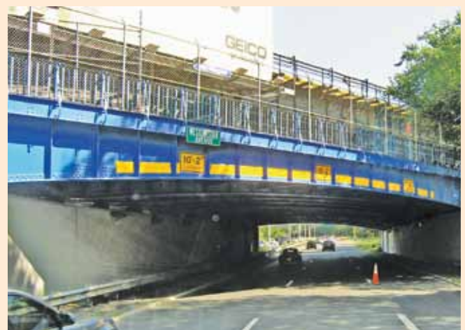
Retro-reflective material installed on Westchester Avenue bridge over the northbound Hutchinson River Parkway.
