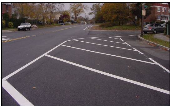
Roadway markings were utilized to improve geometry of roadway, narrow the roadway into one travel lane and provide parking
