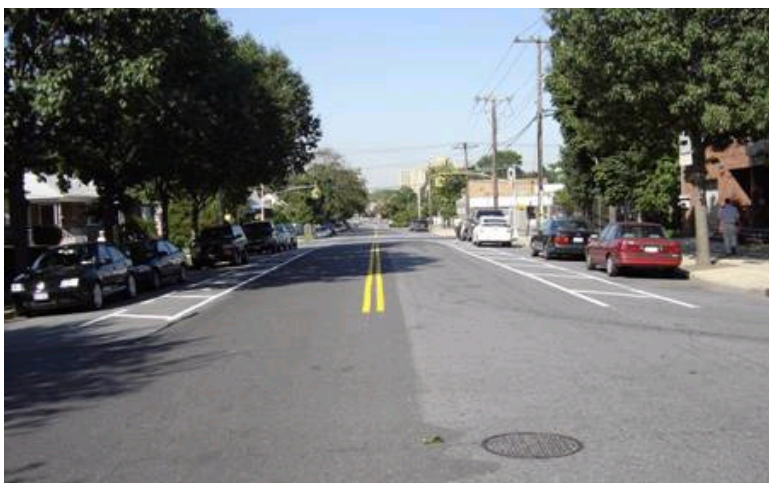
Roadway markings effectively narrowed 80 th Avenue to one lane in each direction
