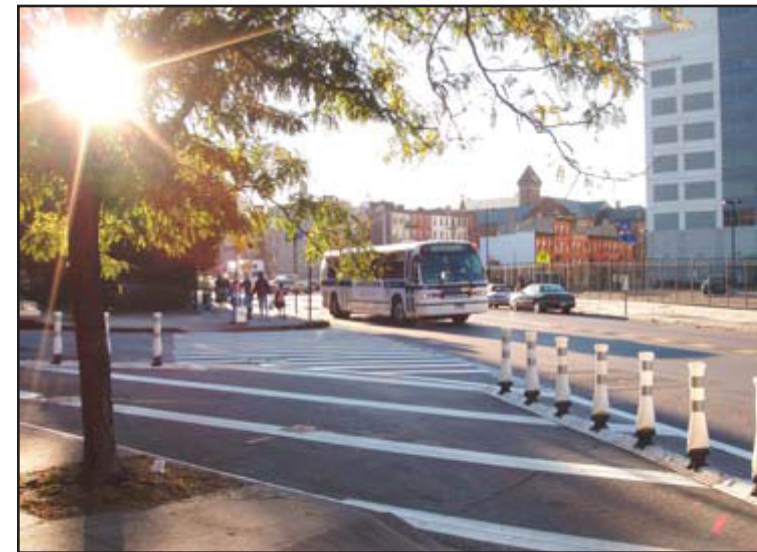
Through the use of flexible bollards and markings, the Department normalized the intersection and significantly shortened the crossing distance across Gates Avenue
