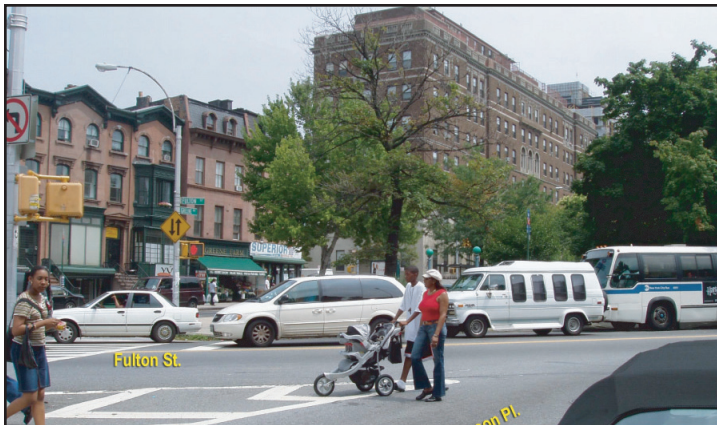
On eastbound Hanson Place approaching Fulton Street, the right-turn slip created difficult, unprotected crossing for pedestrians
