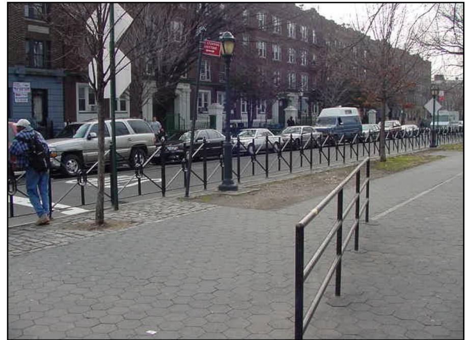
Pedestrian barriers along the service road island prevent individuals from crossing the service road midblock
