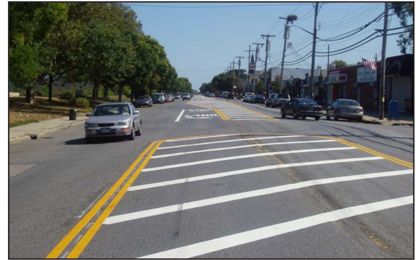
New painted center median and turning bays
