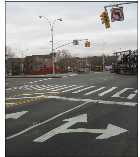
New markings and signage were installed to improve safety and operation of the intersection
