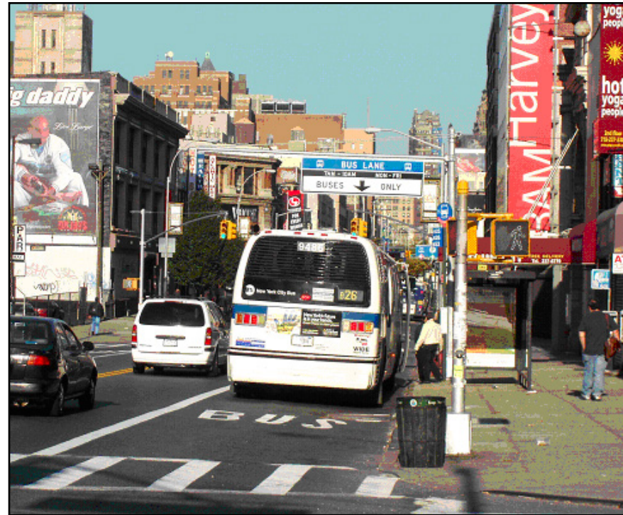
Dedicated bus lanes and newly designed overhead signs were installed to make the bus lanes more prominent.
