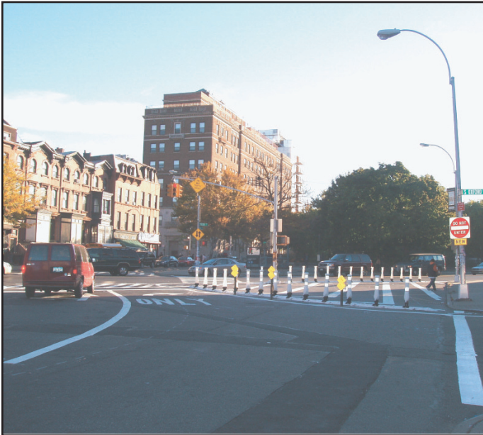
At Hanson Place, the Department eliminated the “free right turn” through the use of markings and flexible bollards, as well as shortening the crossing distance by half
