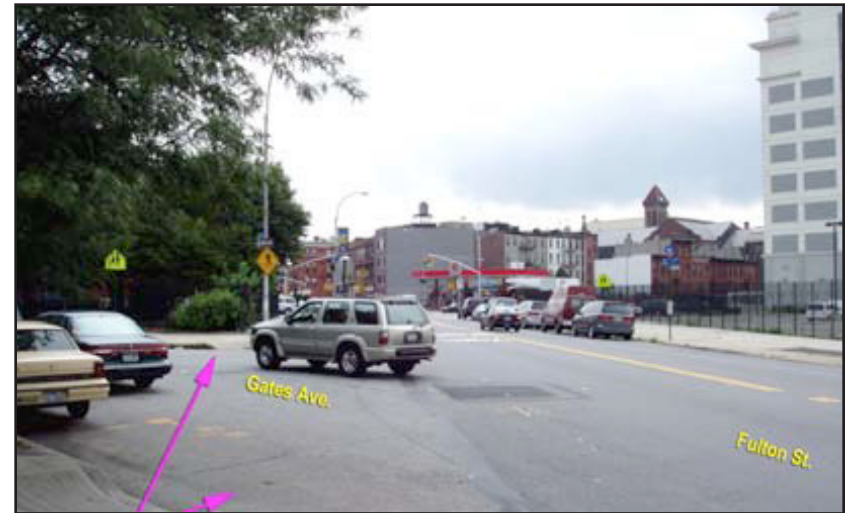
At Gates Avenue and Fulton Street, the offset geometry contributed to speeding, as well as a long crossing for pedestrians
