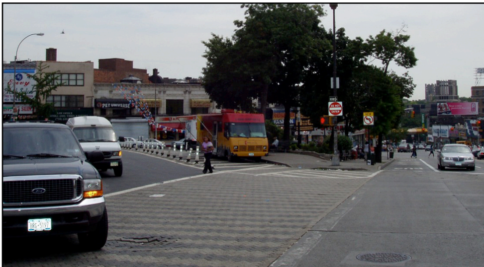
Detailed view of several of the improvements including one-way conversion of slip ramp, modified neckdown and flexible delineators surrounding the park
