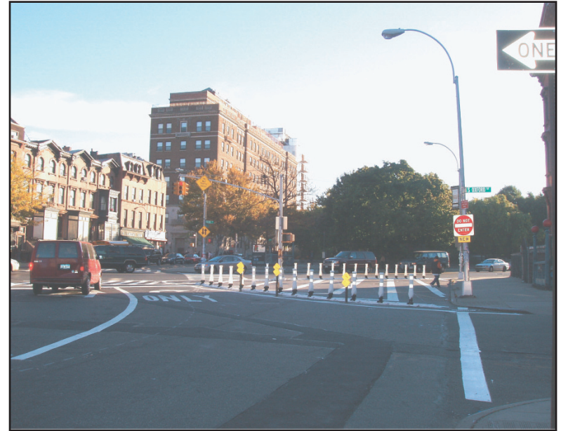
At Hanson Street, the Department eliminated the “free right turn” through the use of markings and flexible bollards, as well as shortening the crossing distance by half
