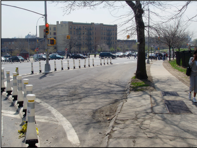
Detailed view of additional pedestrian space created by the use of curb mounted delineators and markings
