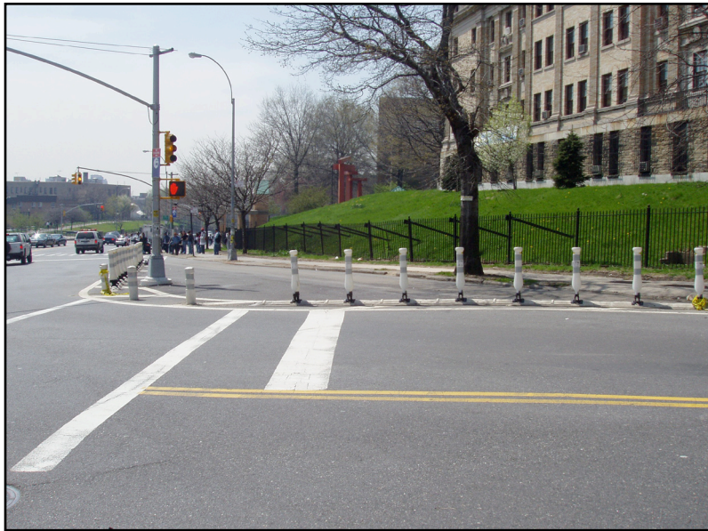
Detailed view of additional pedestrian space created by the use of curb mounted delineators and markings
